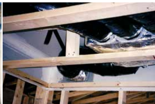
Photograph 9: More Dropped Ceiling – The returns are "passive" – transfer grilles into the dropped ceiling and a large ceiling register in the corridor dropped ceiling connecting the dropped ceiling to the corridor. The supplies are "active" hard ducted.
