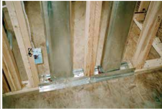
Left – Photograph 1: High Supply Registers – As window thermal performance improved, we learned to “throw” the air across the room from registers located high on interior walls. Centre – Photograph 2: Small Ducts – Better windows also meant smaller ducts. Ducts could easily fit in interior walls. Right – Photograph 3: No Short Circuiting – The supply duct and the return duct could be located up high on the same wall a couple of feet apart.
