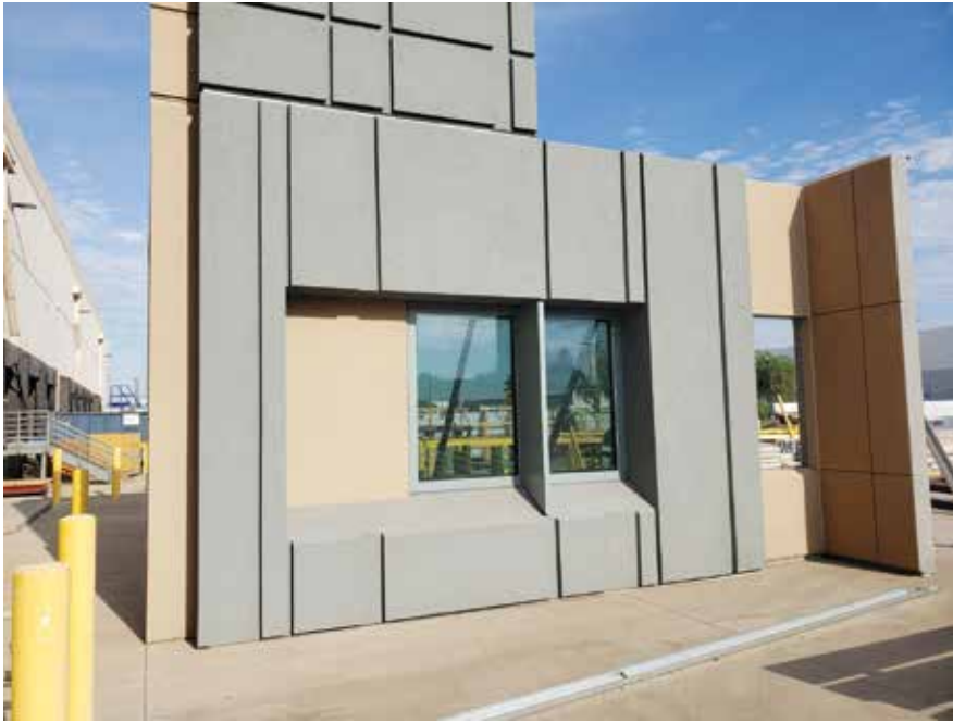
Figure 7: Mockup that includes several typical panel details and aesthetic components for review.
