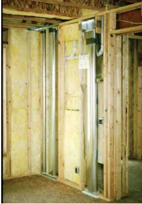
Left – Photograph 1: High Supply Registers – As window thermal performance improved, we learned to “throw” the air across the room from registers located high on interior walls. Centre – Photograph 2: Small Ducts – Better windows also meant smaller ducts. Ducts could easily fit in interior walls. Right – Photograph 3: No Short Circuiting – The supply duct and the return duct could be located up high on the same wall a couple of feet apart.
