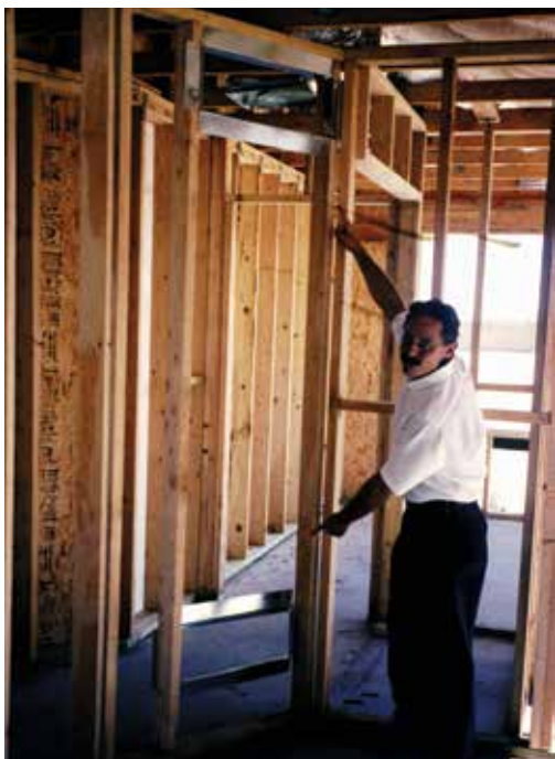
Left – Photograph 4: Transfer Grilles – Grille high on one side, low on the opposite side to control light and noise transfer.
