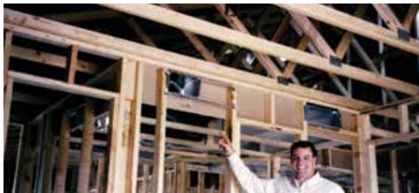
Above – Photograph 10: Still More Dropped Ceiling – The supply grilles and return grilles share the same wall. Right – Photograph 11: Fabulous Windows – With “fabulous” windows we can get rid of the supply return ducts all together. Having said that, we will still need some means of distributing ventilation air. Fully ducted HRVs and ERVs are more than up to the task. Far right – Photograph 12: Lousy Windows – “Dehumidifiers” that prevented high levels of interior moisture.
