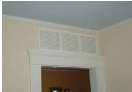
Left – Photograph 4: Transfer Grilles – Grille high on one side, low on the opposite side to control light and noise transfer.
