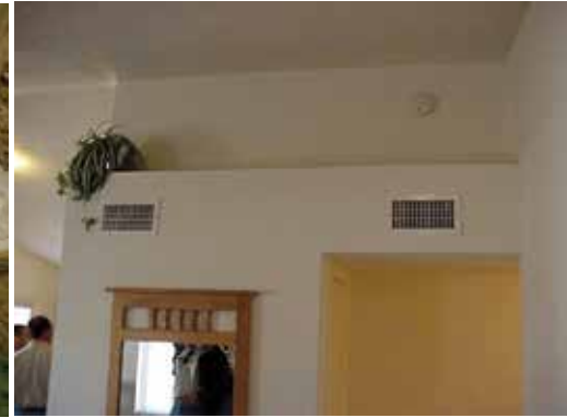
Left – Photograph 1: High Supply Registers – As window thermal performance improved, we learned to “throw” the air across the room from registers located high on interior walls. Centre – Photograph 2: Small Ducts – Better windows also meant smaller ducts. Ducts could easily fit in interior walls. Right – Photograph 3: No Short Circuiting – The supply duct and the return duct could be located up high on the same wall a couple of feet apart.
