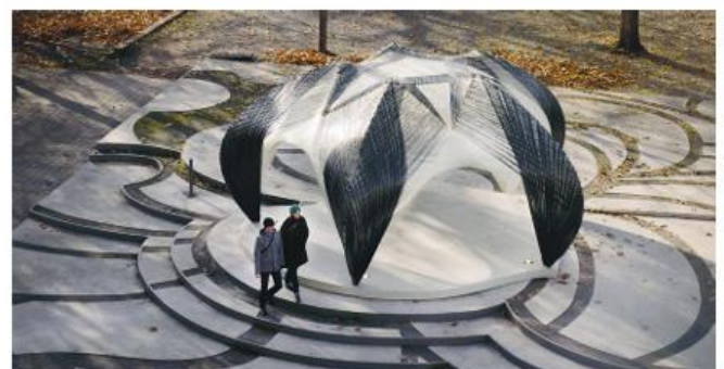
The Institute for Computational Design (ICD) and the Institute of Building Structures and Structural Design (ITKE) at the University of Stuttgart have completed a research pavilion that is entirely robotically fabricated from carbon and glass fibre composites.
