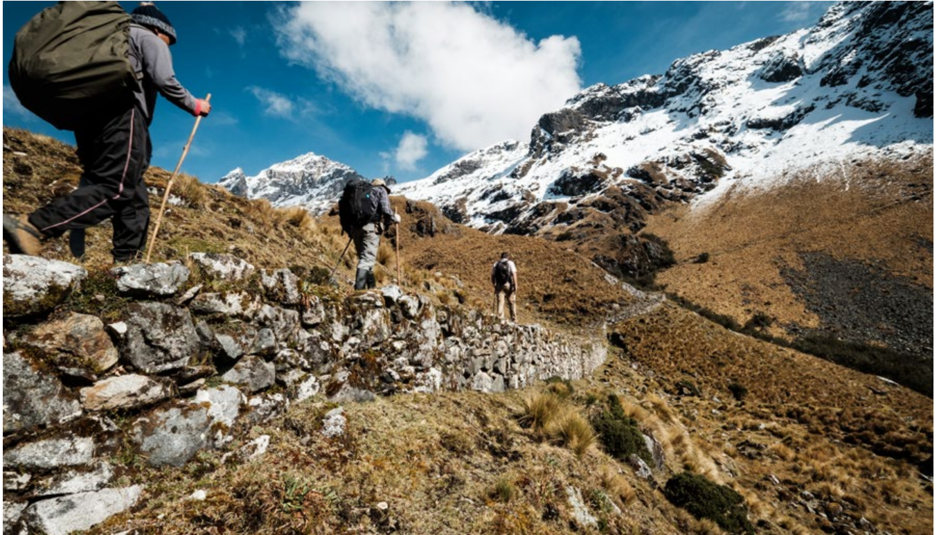
The Inca road as it approaches the high pass at Choquetecarpo.
