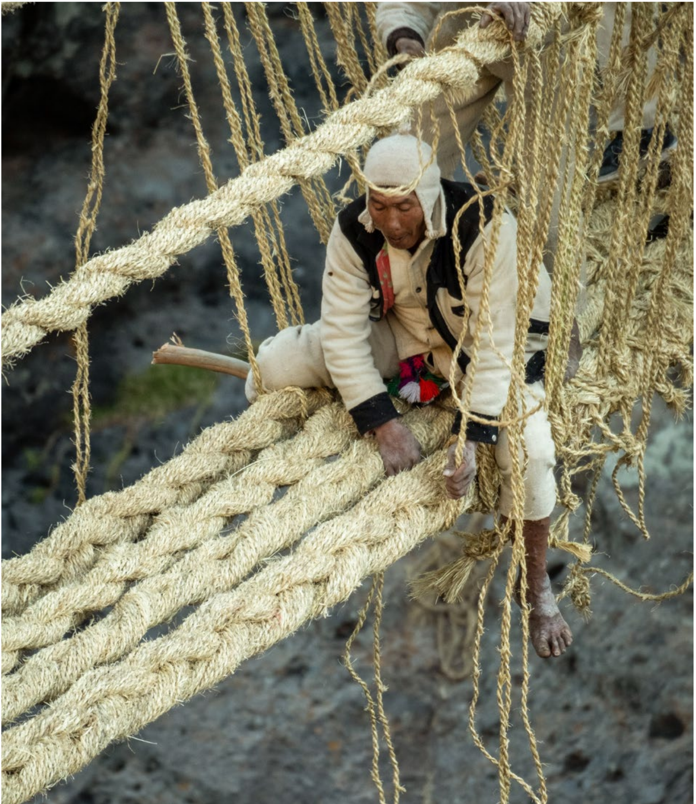
Bridge building at Q'eswachaca.
