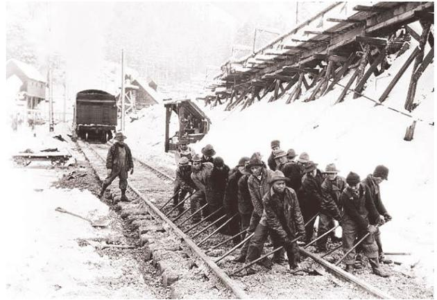
Photograph of Chinese American railway workers straightening track in the construction of the Cascade Tunnel ca. 1928.
