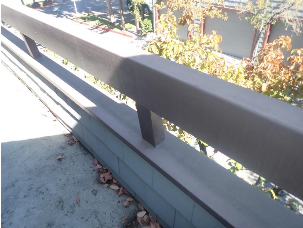
Figure 51. Guardrail that is more flexible than typical.
