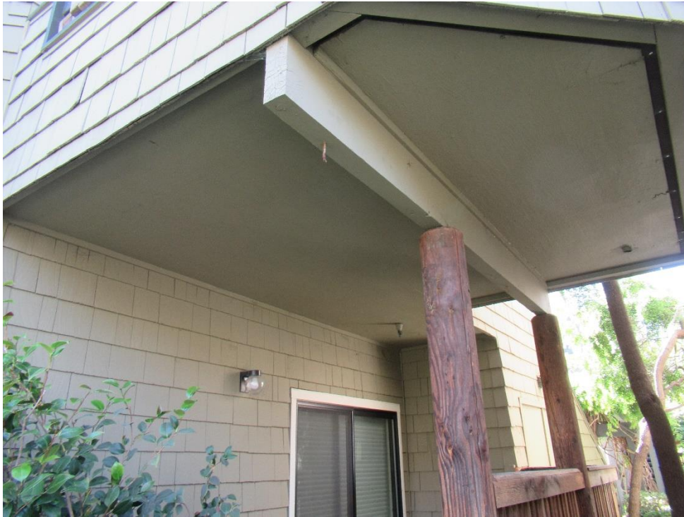
Figure 18. Unit deck with concealed framing.
