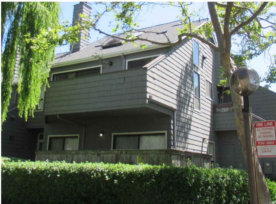
Figure 17. Unit deck with concealed framing.
