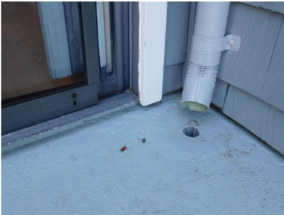
Figure 25. Downspout to roof than drains onto second floor deck.
