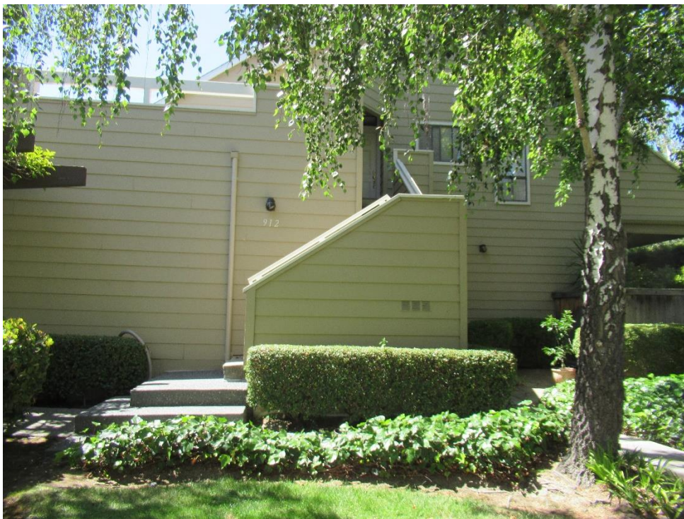
Figure 8. Entry stairs and deck at condominium-type street-side building.
