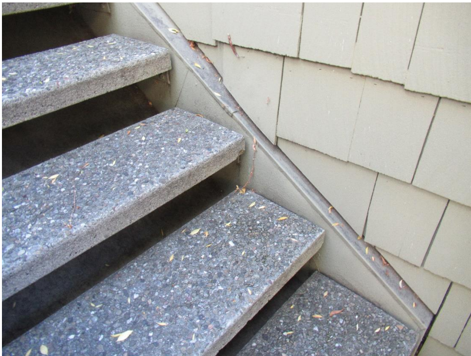
Figure 56. Stair stringer covered with sheet metal cladding.
