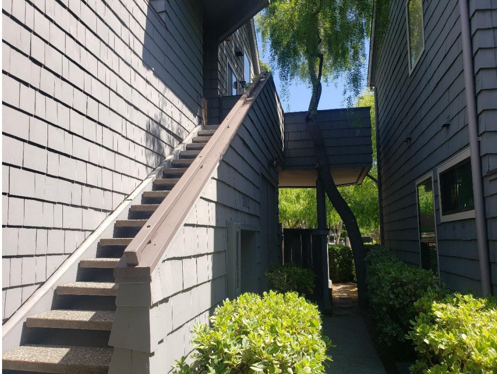
Figure 53. Back stair at street-side building.
