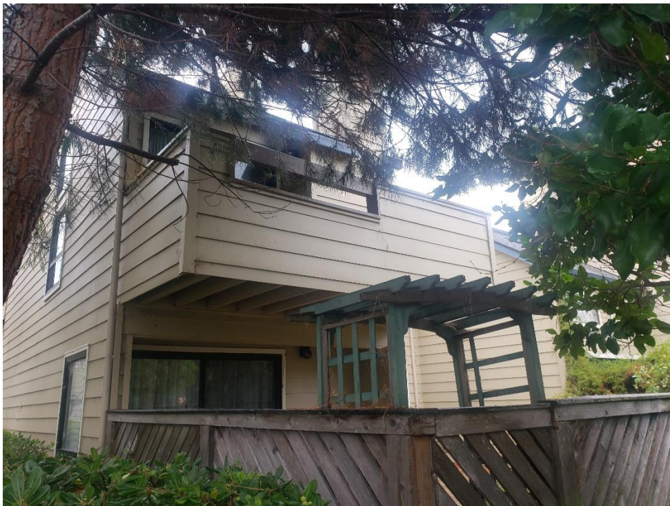
Figure 34. Deck with exposed framing.
