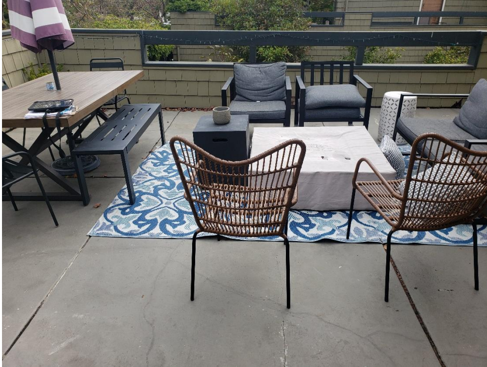
Figure 43. Unit deck above garage with concrete topping slab.
