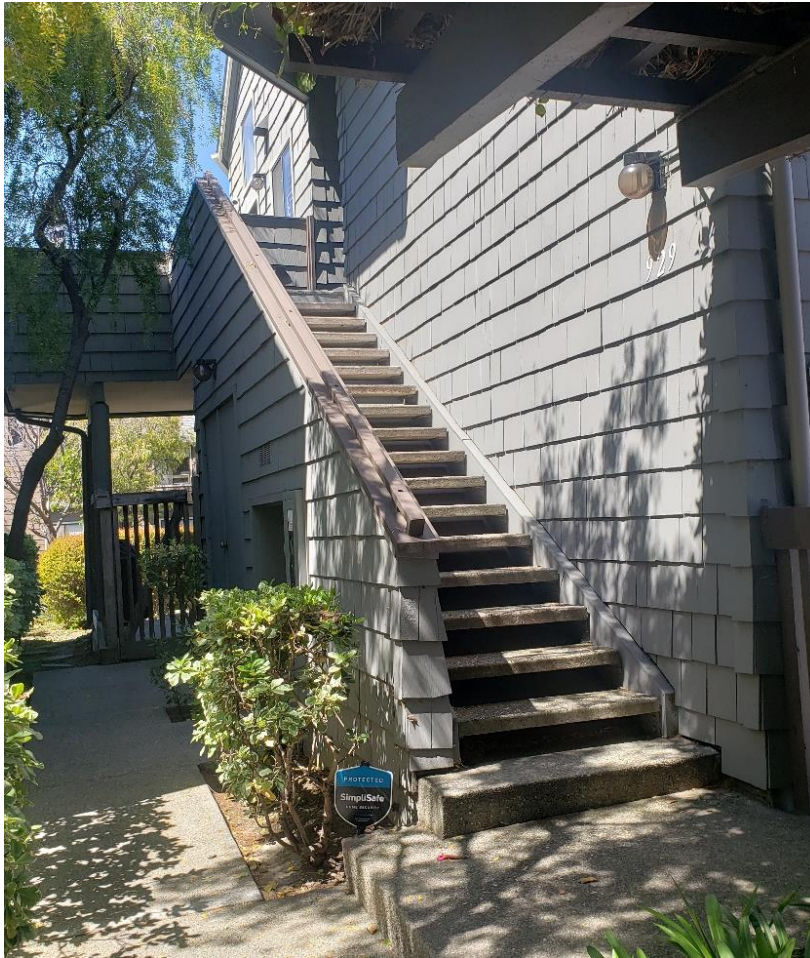
Figure 9. Entry stairs and deck at condominium-type street-side building.
