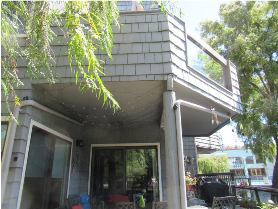
Figure 5. Unit deck not over garage with concealed framing.
