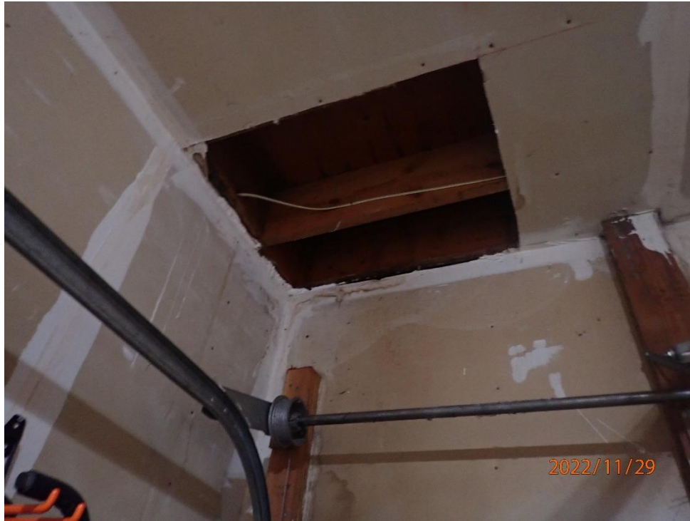
Figure 12. Inspection opening in garage ceiling.
