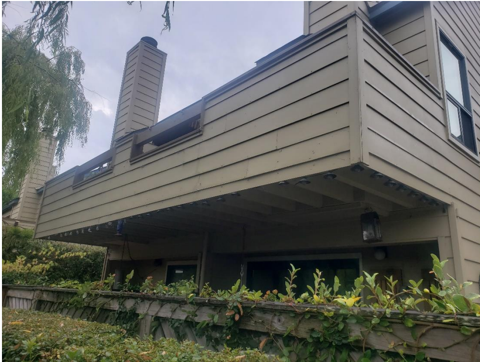
Figure 33. Deck with exposed framing.
