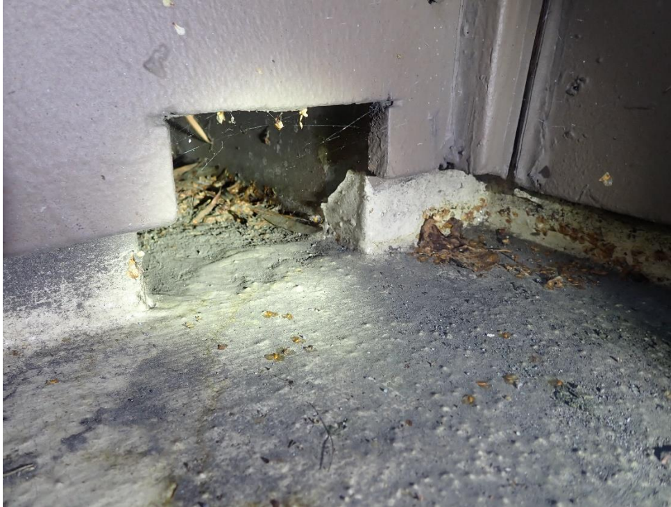
Figure 24. Scupper with reverse slope.
