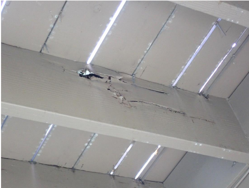
Figure 37. Significant wood decay at exposed deck joist.
