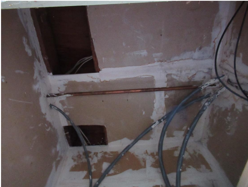
Figure 15. Inspection openings in ceiling of electrical room.
