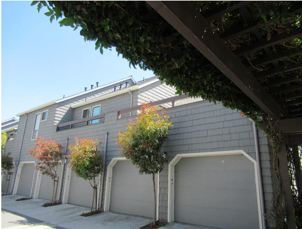
Figure 7. Unit deck over garage.
