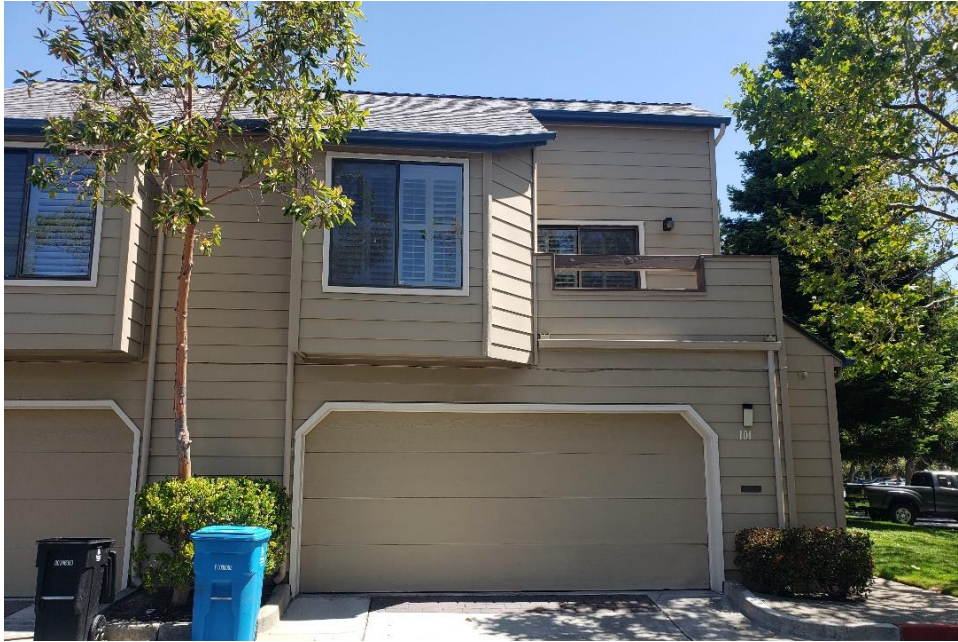
Figure 1. Harbortown townhouse-type building.
