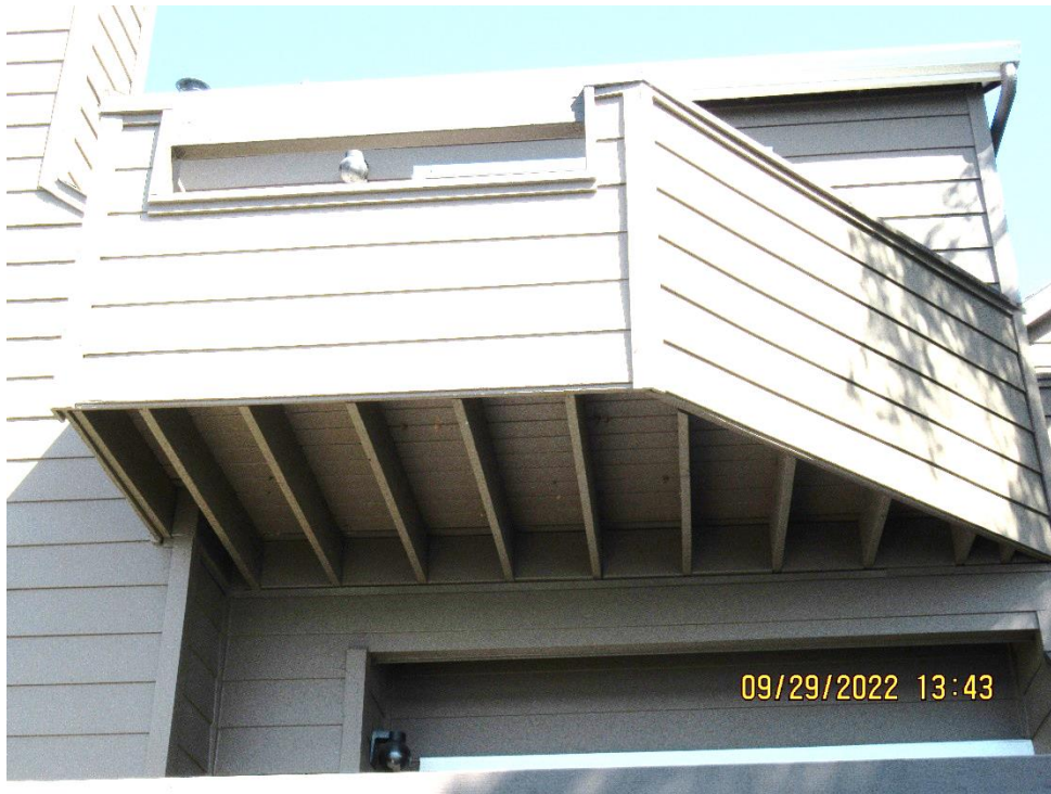
Figure 35. Exposed deck typical framing.
