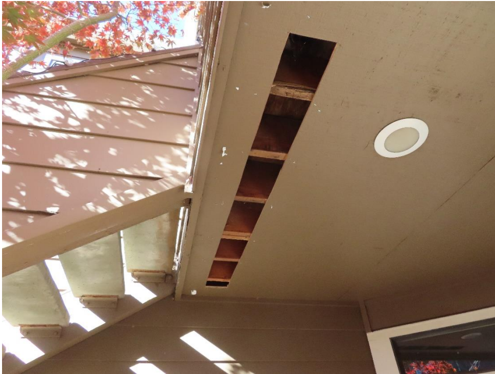
Figure 16. Inspection openings in entry deck ceiling soffits.
