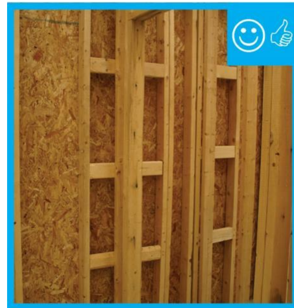
Ladder blocking to fit insulation behind studs
