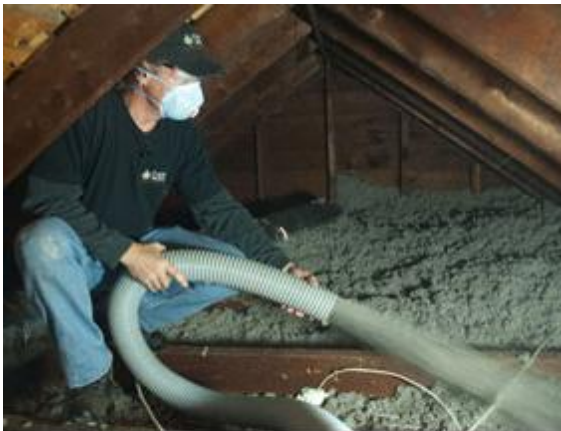
Blowing cellulose insulation to R-49 in attic
