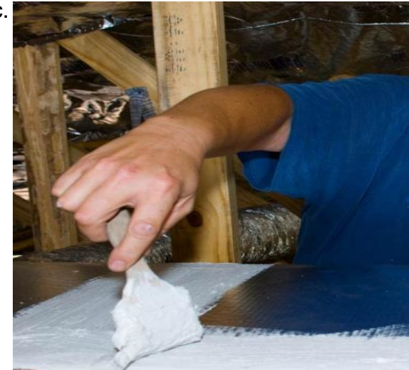
Duct Quality Insulation: Duct Mastic
