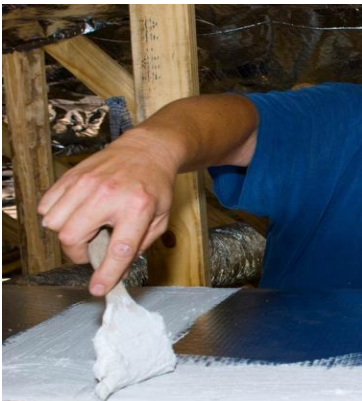
Quality Duct Installation: Duct Mastic
