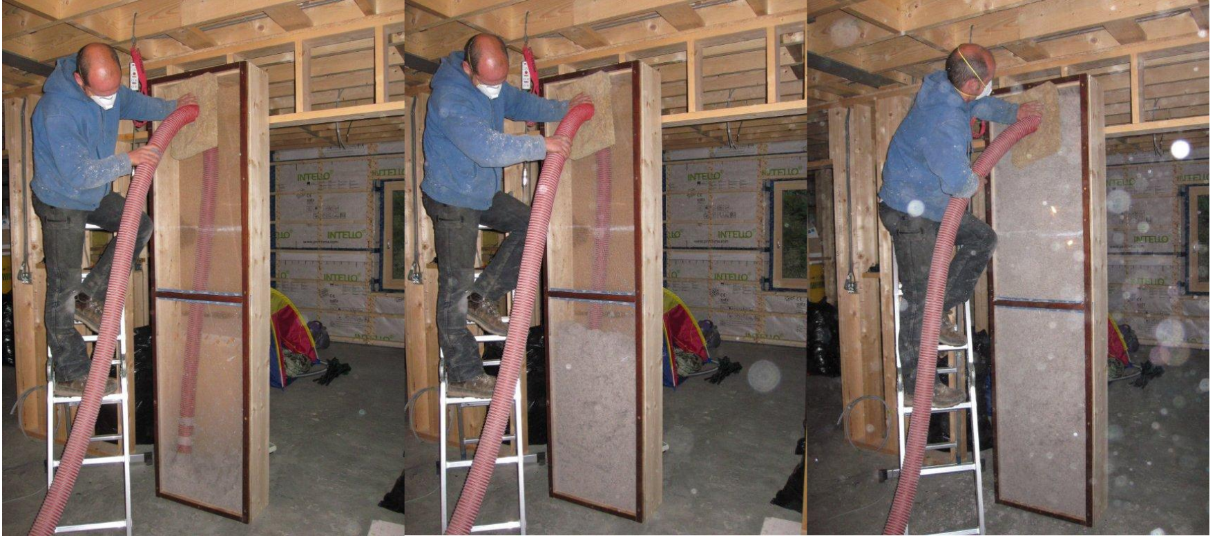
Blown-in cellulose, quality insulation installation
