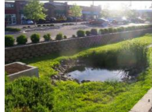
Detention ponds with filtration plants can help the water as it enters, sending clean water to the underground aquifer.
