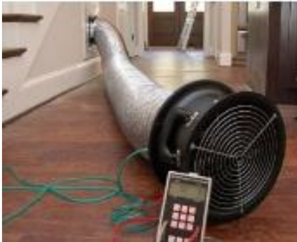
HERS Duct Blaster Test
