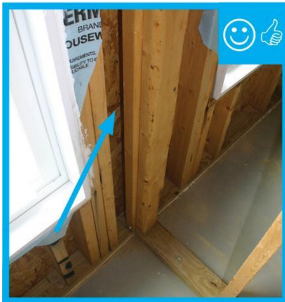
1" gap to slip insulation behind stud
