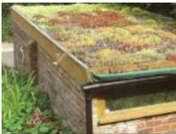
Living roofs absorb rainwater, reducing the amount of runoff from a building. They require structural reinforcements and a super sealed moisture barrier.
