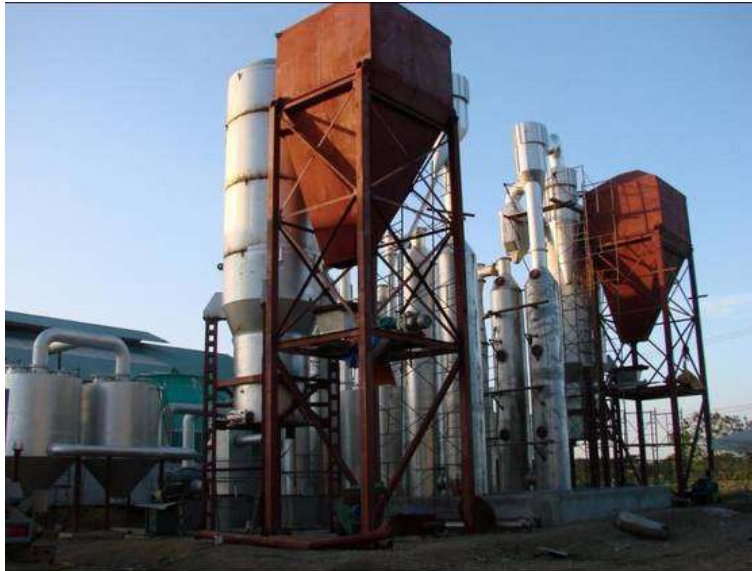
Figure 5: 1.2 MW Fengyu biomass generator in China
