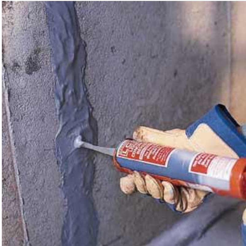
Solution: Epoxy injection
