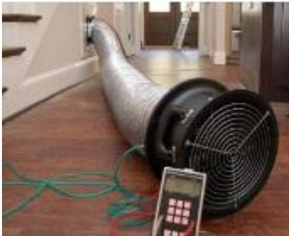
HERS Duct Blaster Test
