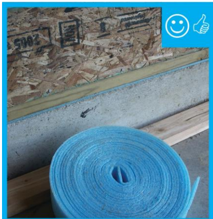
Sealed above-grade sill plates
