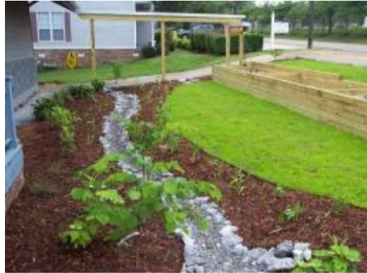
Bioswales help mitigate flooding by directing the water downhill and are used in place of traditional concrete gutters.
