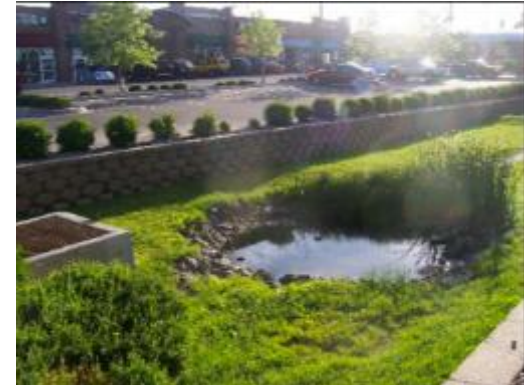
Detention ponds with filtration plants can help the water as it enters, sending clean water to the underground aquifer.
