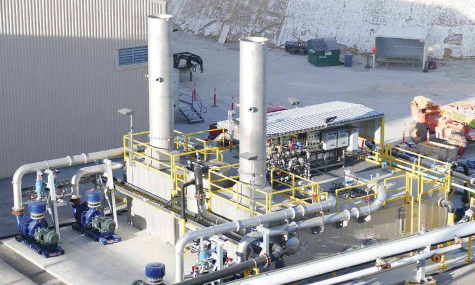
A 60 MM Btu/h SubCom® direct-fired process water heater for Sulphate of Potash production from Great Salt Lake Brine in Ogden, Utah.
