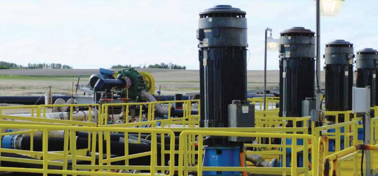
A 182 MM Btu/h SubCom® unit to heat a potash solution mining brine in Patience Lake in Saskatchewan.
