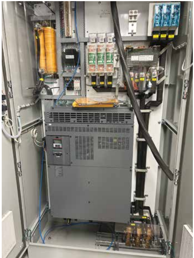
In 2025, JA Tech executed a VFD upgrade at a local potash mine.
