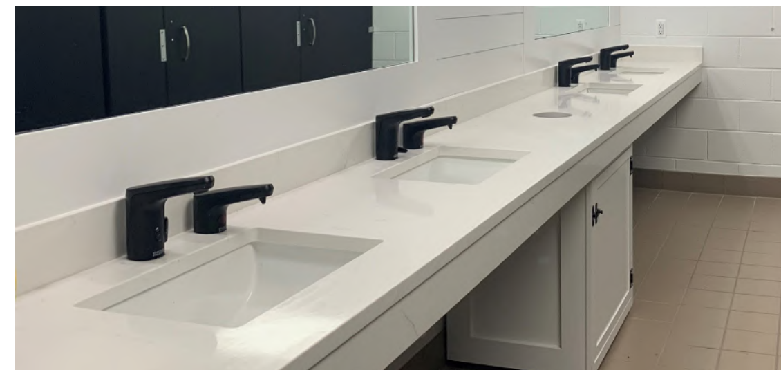
Northpointe Christian Schools in Grand Rapids, Michigan wanted an upscale look for their new restroom renovation. They selected the E-Tronic 80 touchless faucet and soap dispenser in matte black because it is both easy to maintain, as well as stylish for a modern look. The E-Tronic 80 has easy to access above-deck electronics, integrated ASSE 1070 certified scald protection, optional user adjustable temperature control and is easy to adjust and monitor with the CF Connect app. It is the ultimate in restroom hygiene, convenience, and reliability.
