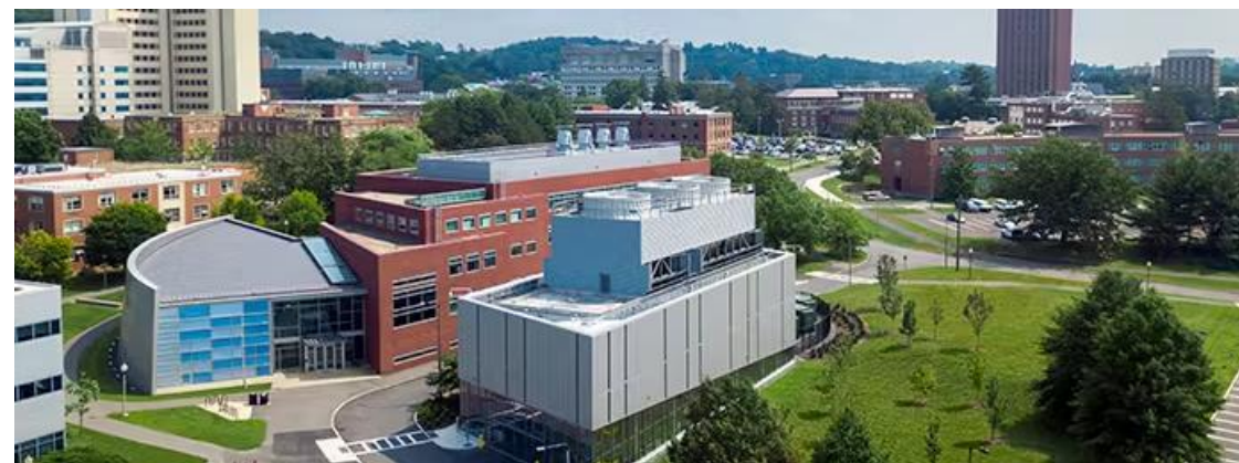
University of Massachusetts Amherst North Chiller Plant
