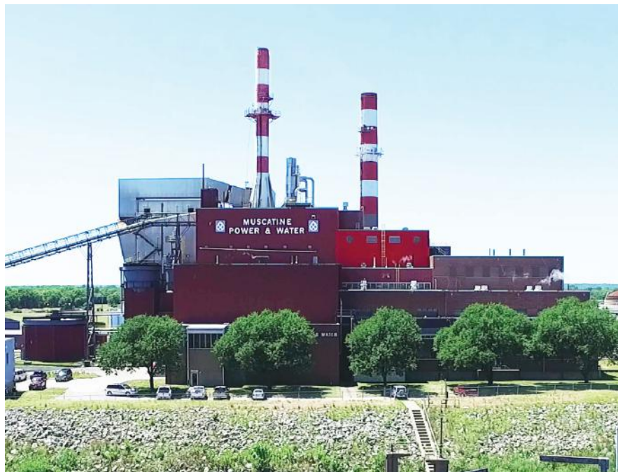
Plant 1 houses Units 7 and 8 will continue to operate as peaking units in 2023.
