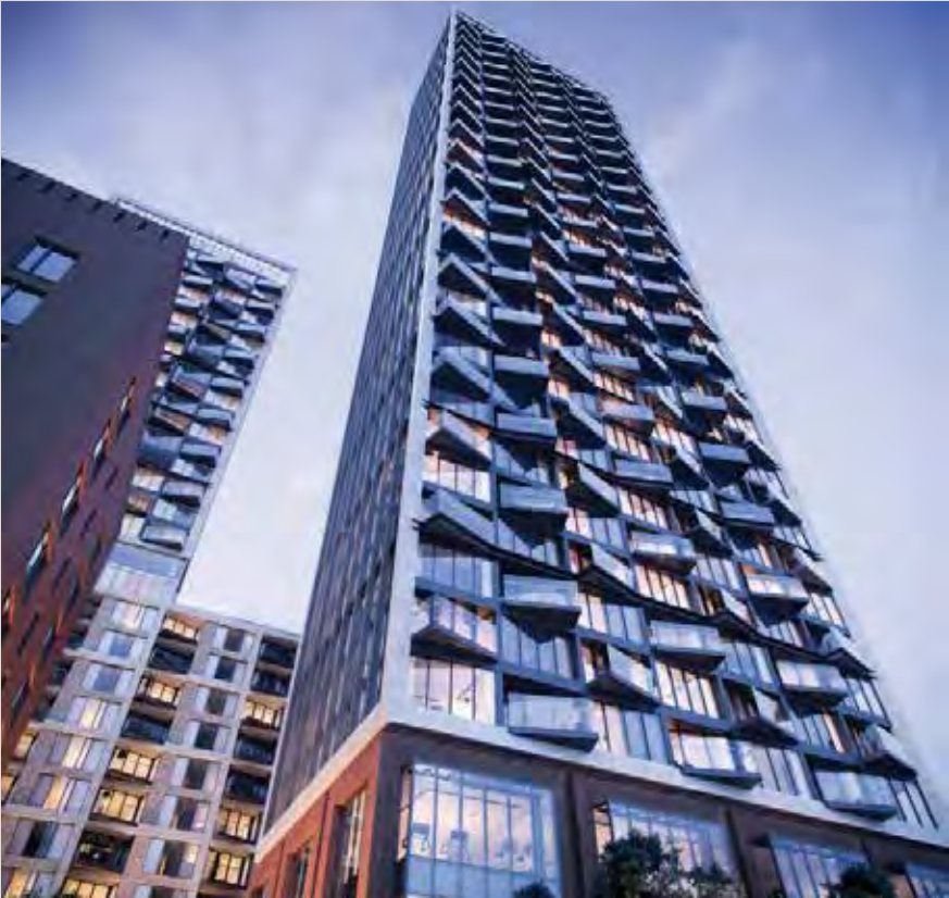
Portal West, LONDON, UK
