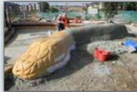
First Coat of Paint being applied - Image 3
