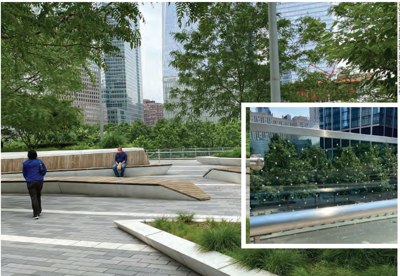
Birds flying across Liberty Park collided with its glass railing as they attempted to reach the greenery beyond. Feather-friendly’s dot pattern makes the glass visible as an obstacle to even the smallest of birds, allowing them to avoid it.
