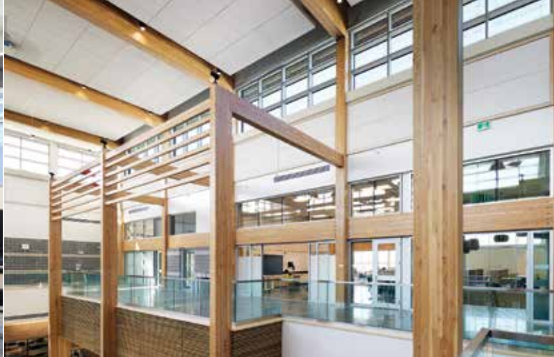
Construction of the 16,224 square meter, two-storey facility began in December 2020 and was completed on budget and on time in July 2023.
