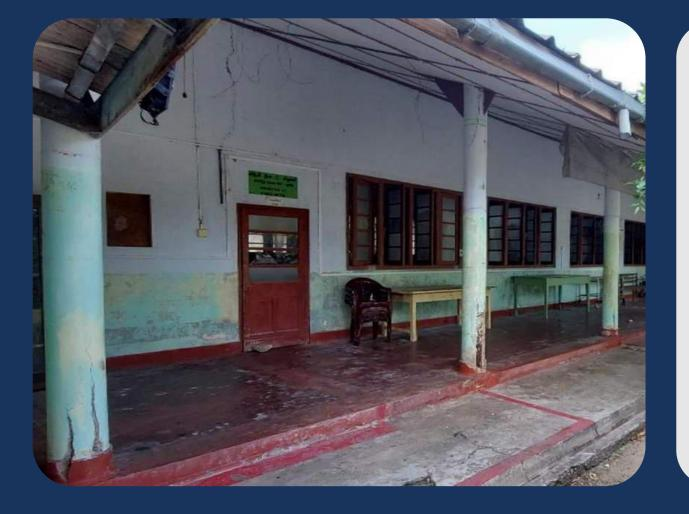
Structurally, the current paediatric ward is in bad shape and the fabric of the building is in poor condition. The roof and the pillars holding it up, are a cause for concern.
