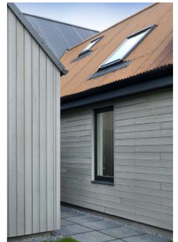
Russwood SILA Select® cladding factory coated in SiOO:X Mid Grey, Fiddes Architects
