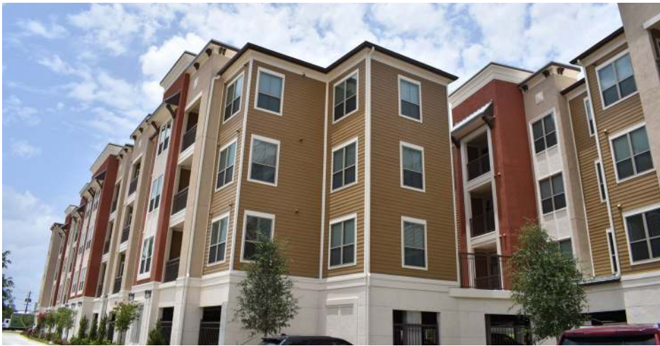
Somerset Lofts will bring 120 new state-of-the-art apartments to Timbergrove, an expanding neighborhood where affordable homes are difficult to find. These homes are a great example of the importance of equitably distributing apartment homes.
