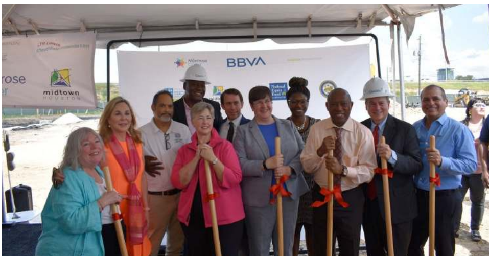
Mayor Sylvester Turner (third from right), former Mayor Anise Parker (fourth from left), and HCDD Director Tom McCasland (center) help break ground on Law Harrington Senior Living Center. This community will be the largest LGBTQ-affirming senior center in the U.S.A., offering 112 affordable apartment homes to seniors. A partnership with the Montrose Center will provide social services and community support to residents.
