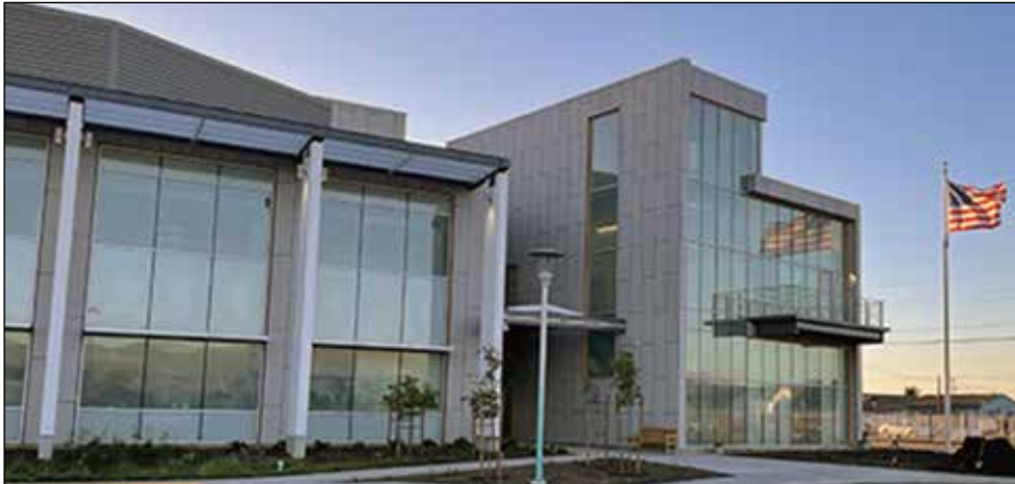
The newly constructed Sam Farr United States Crop Improvement and Protection Research Center is located in Salinas, California. The over 117,000-square-foot research center features state-of-the-art laboratories and greenhouses for fruit and vegetable research. (Photo by Bill Wintermantel, ARS)
