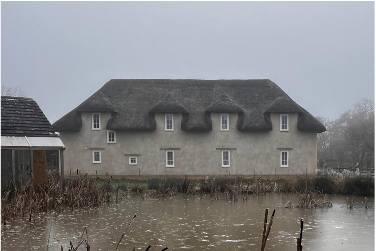
THE FAMILY COB HOUSE, BUILT FROM TRIAL AND ERROR, CONSTRUCTED ENTIRELY OF NATURAL MATERIALS MOSTLY DRAWN FROM THE FARM
