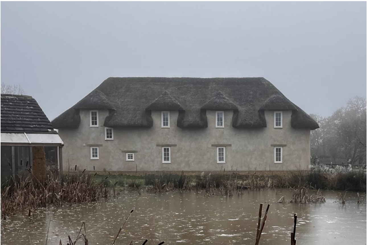
THE FAMILY COB HOUSE, BUILT FROM TRIAL AND ERROR, CONSTRUCTED ENTIRELY OF NATURAL MATERIALS MOSTLY DRAWN FROM THE FARM
