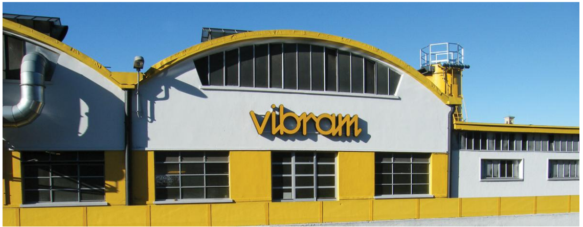
VIBRAM HEADQUARTERS—ALBIZZATE, ITALY
