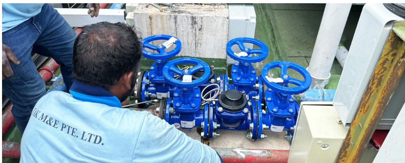
Installation of Norika water meter at StorHub
