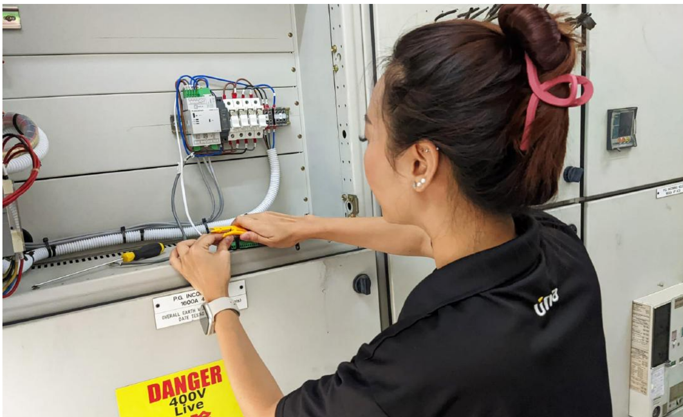
Installation of Socomec electrical meter at StorHub
