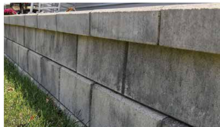
AB Metro Cap designed with overhang, perfect to accommodate lighting.
