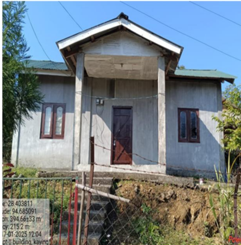
Renovation of SPT II building at Jengging
