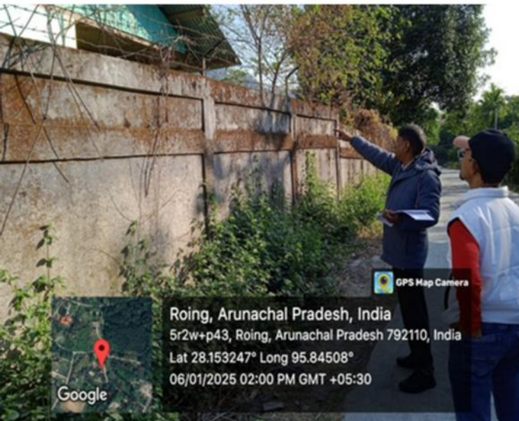
Project Lead inspects the compound wall construction at Arunachal Pradesh Forest Training Institute, Roing
