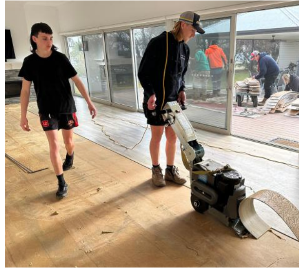
Apprentices remove old floor coverings at Forbes NSW
