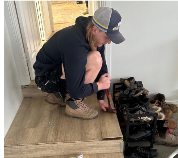
Apprentice removes floor coverings on stairs in Forbes NSW
