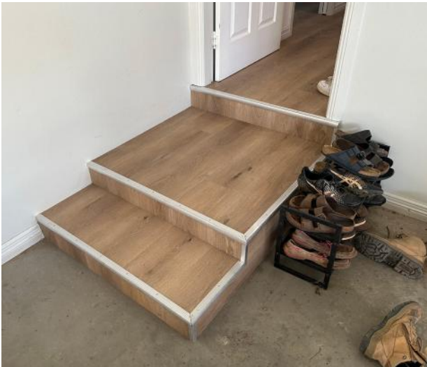
The newly installed flooring on the stairs at Forbes NSW workshop
