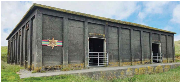
One of the munitions bunkers in Belmont Regional Park.
