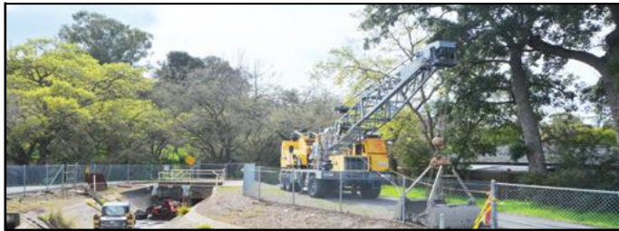
A crane was used to repair the canal
