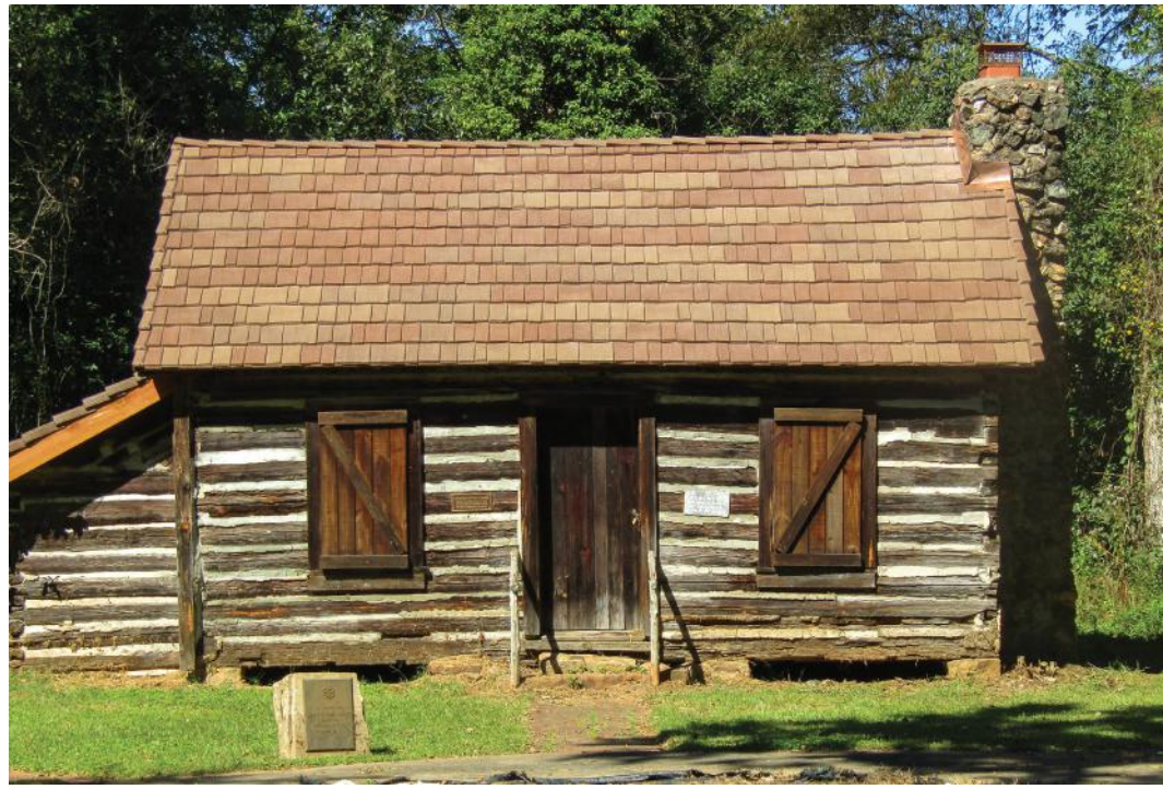
The Fell Cabin in Abbeville has a new roof. (Staff photo by Henry E. Green)
