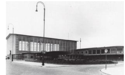
Station Amstel, ca. 1940
