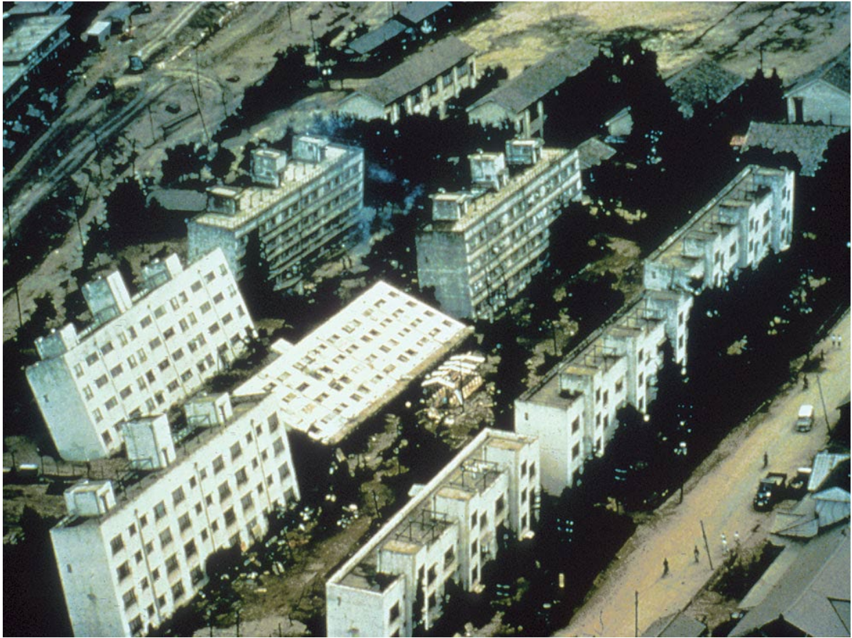
Figure 4.2-9 Liquefaction, Niigata Japan 1964
