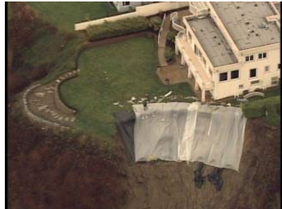
Figure 4.4-2 2007 Northeast Tacoma Landslide
