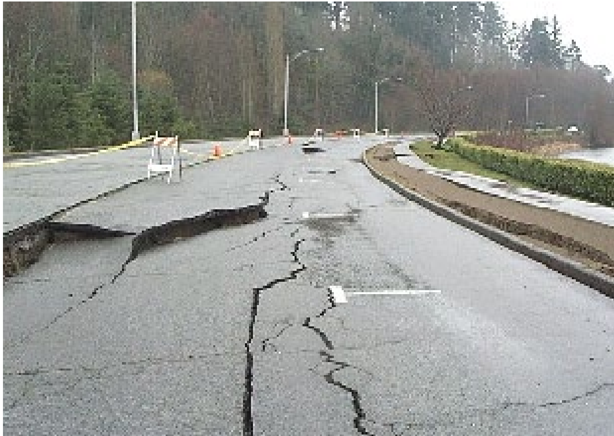
Figure 4.2-10 Lateral Spreading –March 2001
