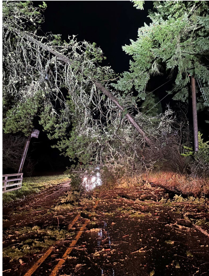
Figure 4.5-1 December 2024 Windstorm Damage
