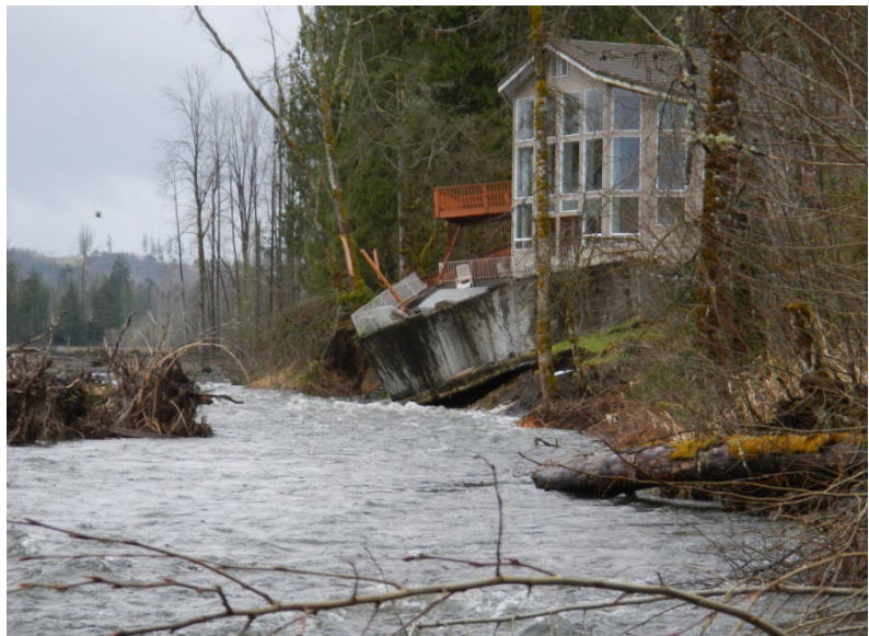
Figure 4.3-2 House Destroyed Due to Erosion from Puyallup River Channel Migration
