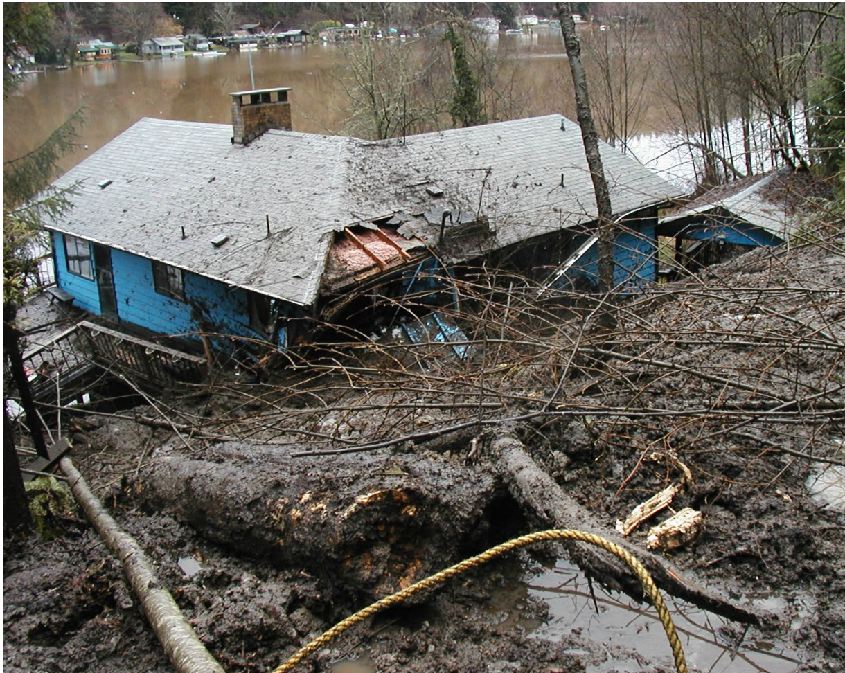
Figure 4.4-5 January 2003 Ski Park Road Landslide
