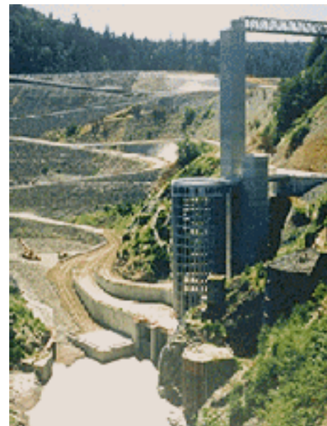
Figure 4.3-2 Mud Mt. Dam Intake 1
