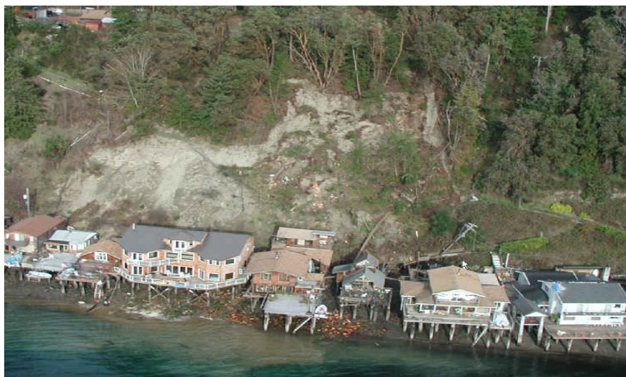
Figure 4.2-8 Salmon Beach, Tacoma – Following February 2001 Earthquake
