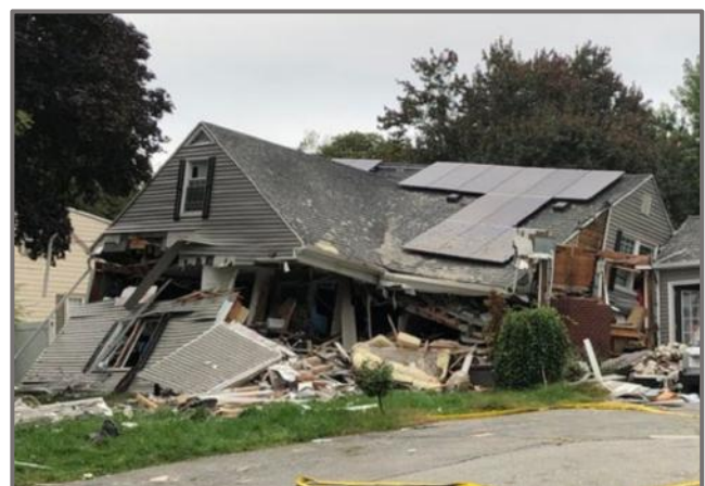
Figure 6: A large home in Lawrence, MA was among the 130 destroyed by gas explosions in 2018 when maintenance workers accidentally over-pressurized the gas main, turning gas-using homes into bombs. All-electric homes are safer. 10
