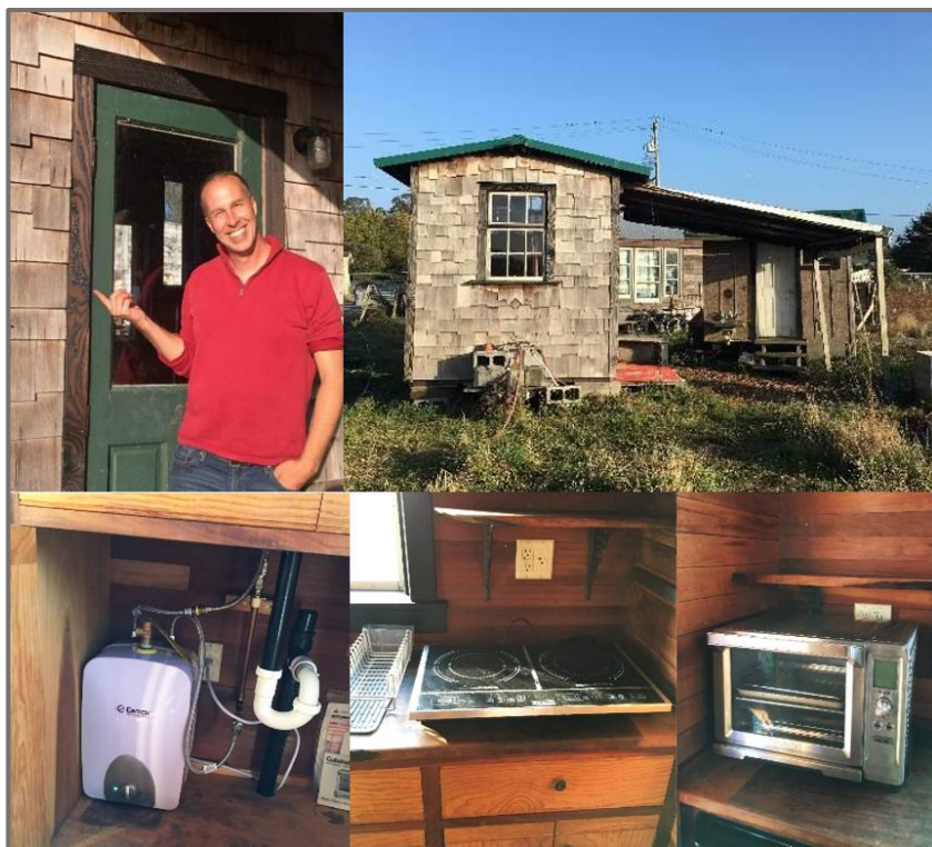
Figure 41: The Power Efficient Tiny Home in Arcata, California on Sean Armstrong’s property—two 1000W water heaters, a 1400W induction cooktop and a 1200W toaster oven and 500W space heater with an ERV keep power demands below 30Amps for both the tiny house and adjacent tiny bathroom.
