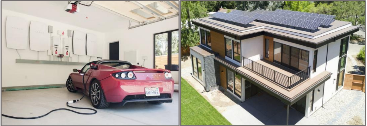
Figure 30: Stanford professor Mark Jacobson's passive house and the four tesla power walls that provide backup power and EV charging.
