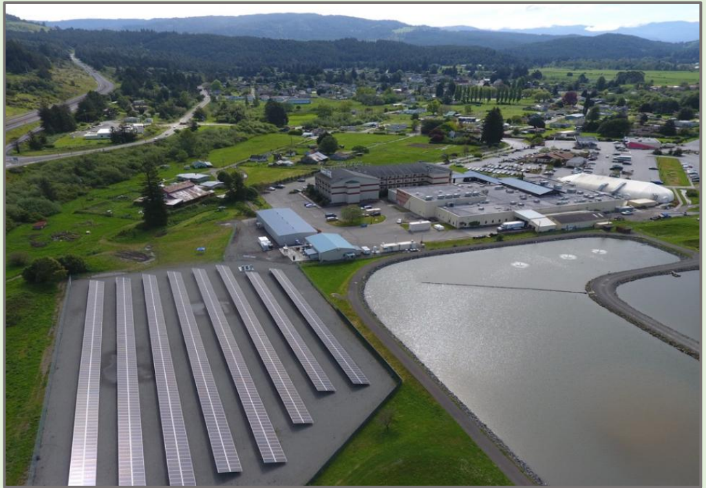
Figure 22: Aerial view of the Blue Lake Rancheria microgrid.
