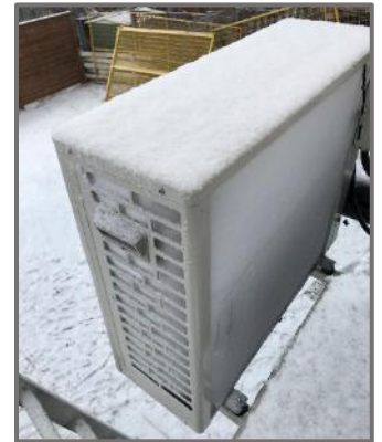
Figure 46: A Sanden CO2 heat pump water heater compressor working outside in 5°F (-15°C) weather. 113
