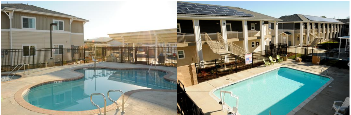
Figure 50: Pacific Companies Zero Net Energy apartment complexes built in 2014 with heat pumps for the hot tub and swimming pools. (left King Station Apartments, King City, CA and right Belle Vista Senior Apartments, Lakeport, CA.)
