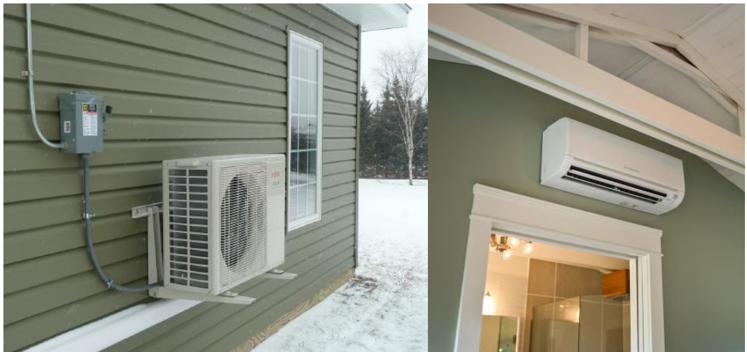
Figure 47: An example of a ductless mini-split heat pump outdoor compressor unit 114 and indoor fan unit 115 .
