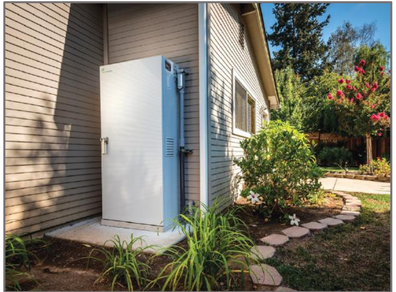
Figure 18: Example of residential battery storage. 59
