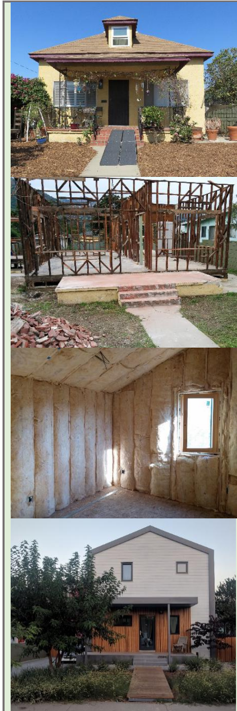
Figure 42: The Perlita Passive House: the beginning, a complete to-the-stud strip, an impressive amount of insulation, and the finished product. 109
