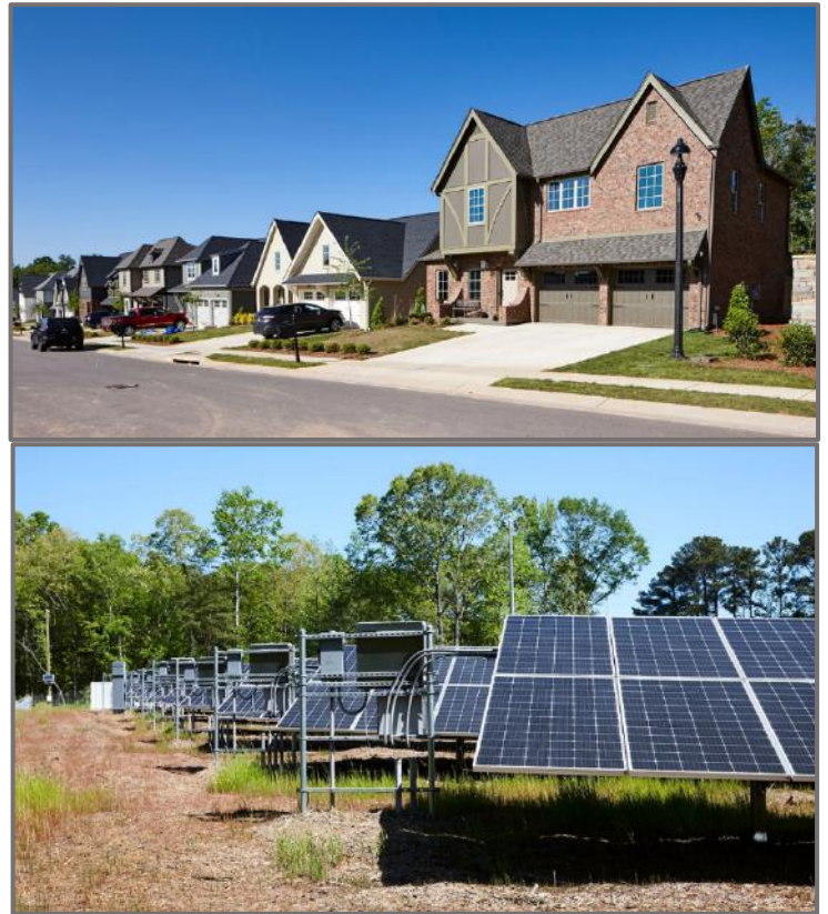
Figure 32: Alabama Power’s Reynolds Landing Smart Neighborhood in Birmingham, Alabama, the housing tract and the solar array. 101
