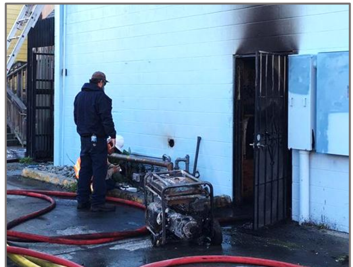
Figure 21: A generator fire broke out in Arcata, CA, during a PSPS in October 2019, resulting in three businesses being temporarily condemned until repairs ensure their safety. 65
