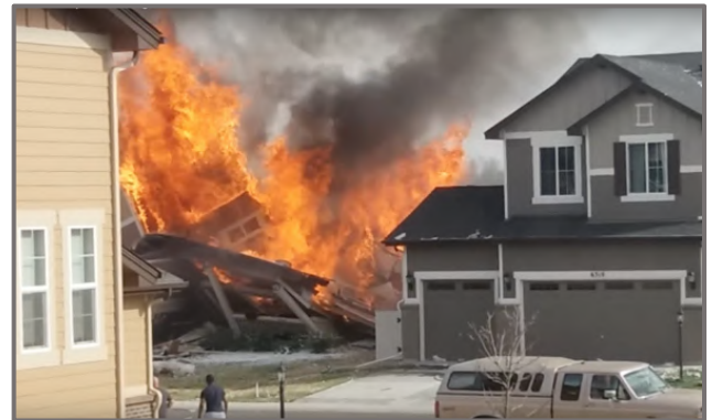
Figure 13: Methane leakage from a Colorado gas well 150' away caused this explosion that killed two brothers. (Photo by CBS)
