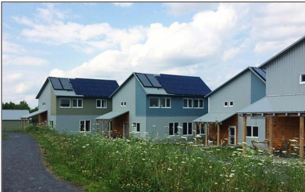
Figure 35: The Third Residential Ecovillage Experience located in Ithaca, New York.
