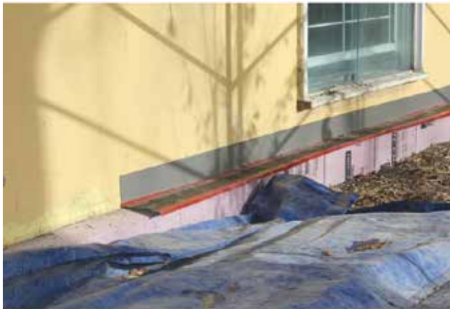
Image 6: Completed below grade insulation of Project 2.
