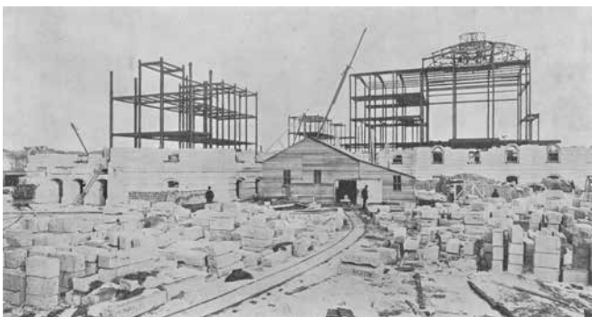
Stone storage and yard on west side of Legislature Building. (Provincial Archives of Alberta, A11027) .
