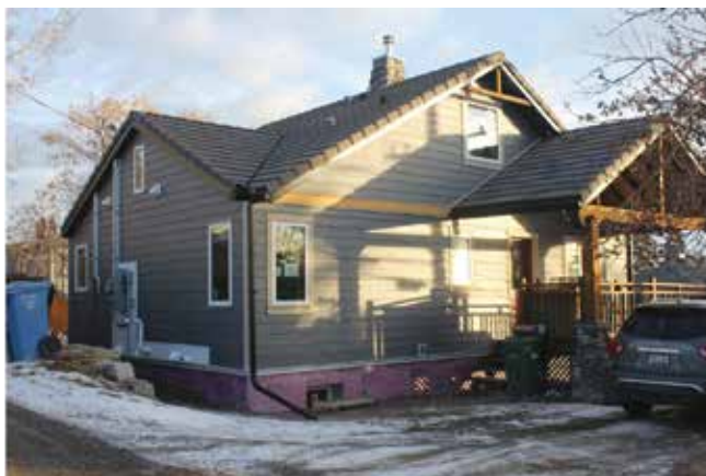
Image 3: Project 1 following completion of retrofit work in 2022.
