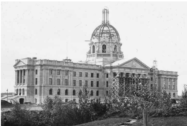
Under construction. (Canadian Museum of History, unknown photographer, 42.13-LS)
