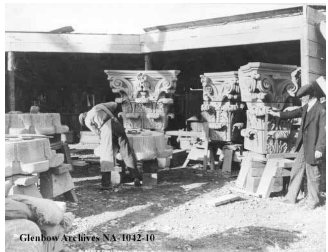
On-site stone fabrication (1911). Allan Jeffers on the right. (Glenbow Museum Archives NA-1042-10).
