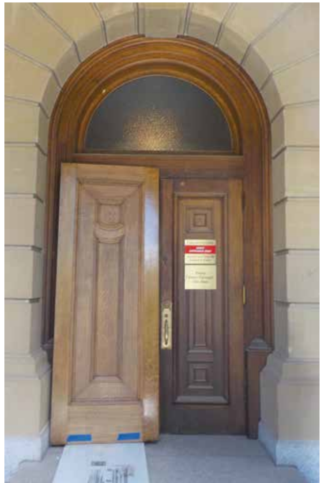
Restored door mockup against existing.
