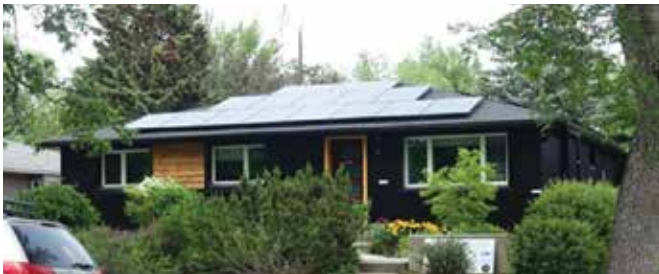
Image 11: Project 3 following completion of retrofit work in 2022.
