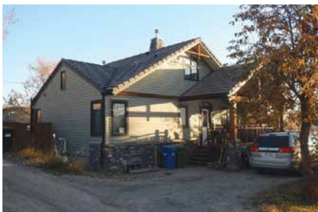
Image 1: Project 1 before retrofit work in 2022.
