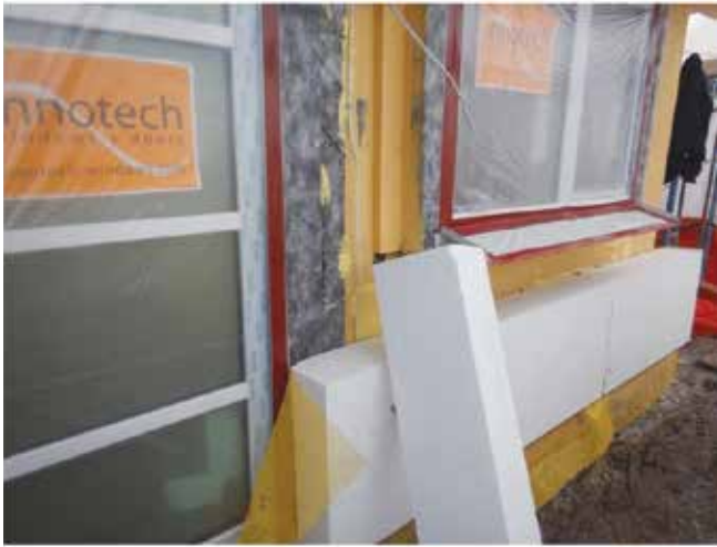
Image 5: EIFS installation in progress around windows on Project 2.
