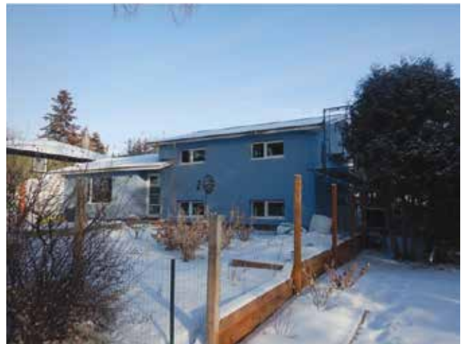
Image 7: Project 2 following completion of retrofit work in 2022.
