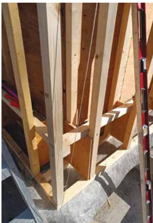
Image 9: Larsen truss framing on Project 3.
