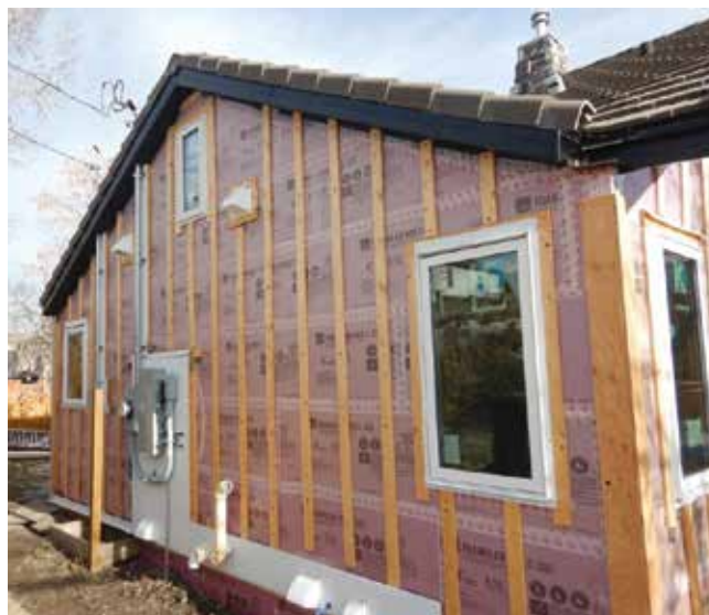
Image 2: Exterior XPS, strapping, and new windows installed on project 1.
