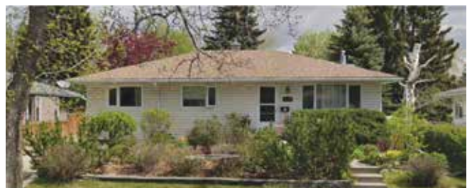
Image 8: Project 3 before retrofit work in 2022
