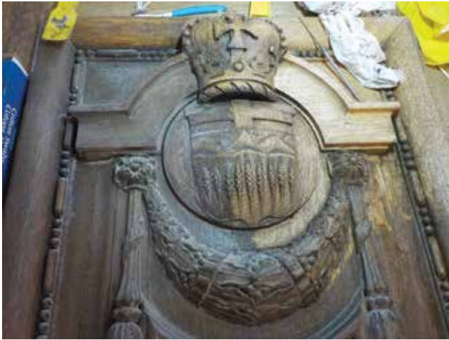
Stripping of existing discoloured stain from north entrance door underway.
