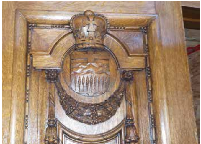
Restored north entrance door.
