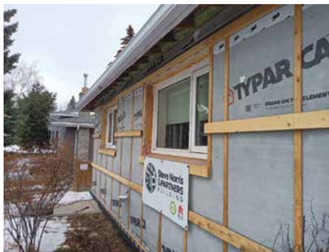
Image 10: Completed Larsen truss assembly of Project 3 with spray foam sealing between wall and attic assemblies.
