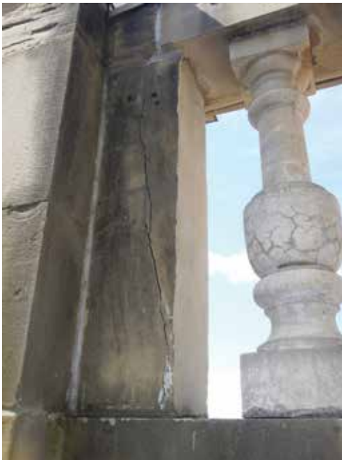
Precast concrete baluster.
