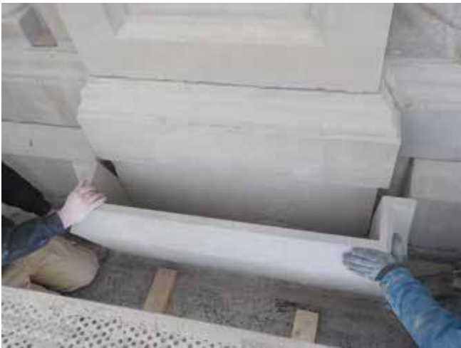
Dry-fit installation of indent repair.
