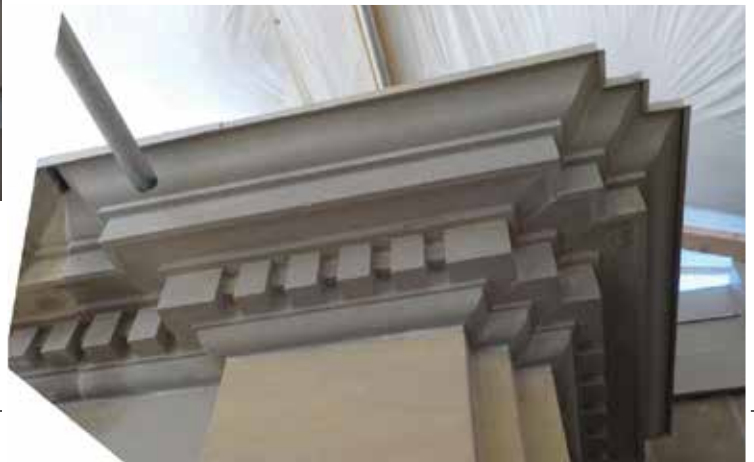
Membrane flashing applied on top of balustrade bottom rail, complete with granules.
