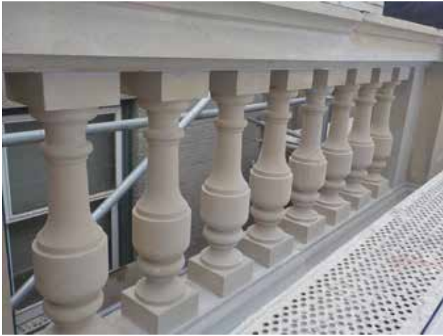
Replacement Paskapoo sandstone balusters.
