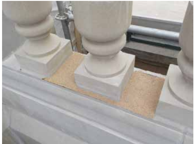
Membrane flashing applied on top of balustrade bottom rail, complete with granules.
