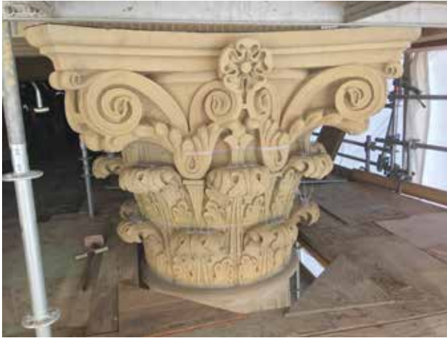
Paskapoo sandstone freestanding column capital during restoration project.
