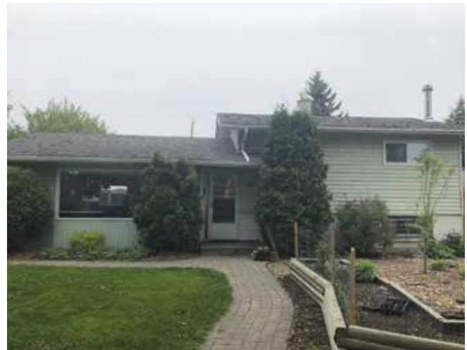
Image 4: Project 2 before retrofit work in 2022.
