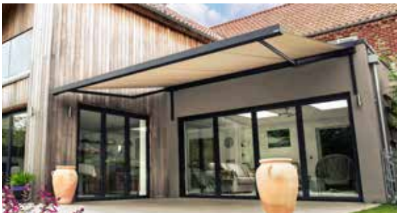
CUBA AWNING ON SPREADER PLATES TO AN EXTENSION
