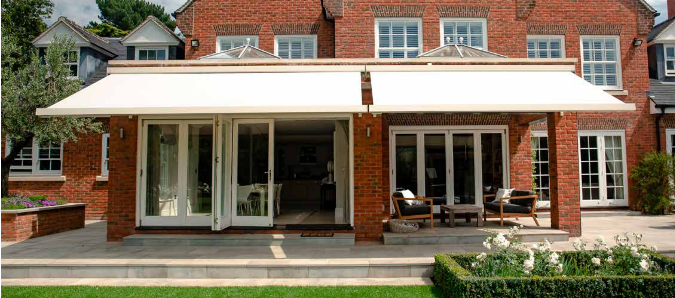
CUBA AWNINGS INSTALLED ON A NEW BUILD PROPERTY
