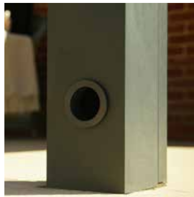
Integrated rain water pipes within the post uprights provide effective evacuation of water from the roof
