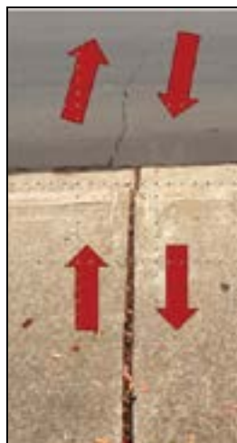
Right-lateral offset curb and sidewalk and cracked pavement on Citrus Circle in the Woodlands east of Oak Grove Road in Walnut Creek (photo M. Steinpress)
