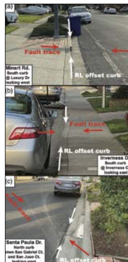
Photographic examples of offset and deflected curbs (white annotations) and evidence of right-lateral shear along the interpreted fault trace (red annotations). Photo locations indicated RL, right lateral. (a) Discrete offset of curbstones on Minert Road, aligned with an echelon cracks in roadway asphalt. (b) Offset and deflection of the south curb and sidewalk of Inverness Drive. (c) Deformation at curb-line and an echelon cracks in road asphalt across Santa Paula Drive. Photos taken by A. Elliott.
