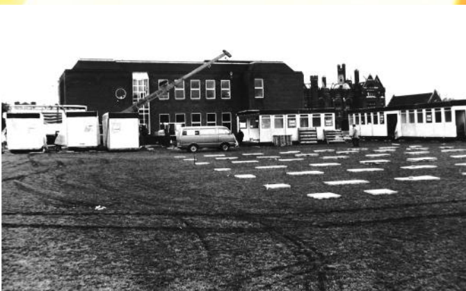
Temporary classrooms on the day they arrived
