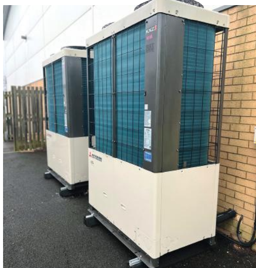
Two MHI KXZ2 Heat Recovery outdoor units were chosen for the project
