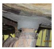
Process kettle developed holes in the weld seam as a result of corrosion. Belzona 1511 used to repair holes for the long term.
