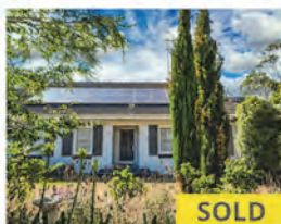
7857 Main South Rd, Second Valley
