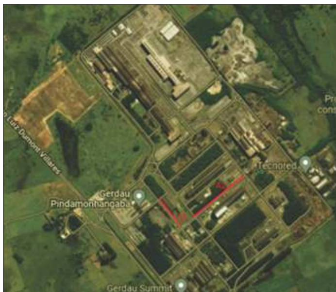
Figure 4: Paint application location in Gerdau Pindamonhangaba plant.
