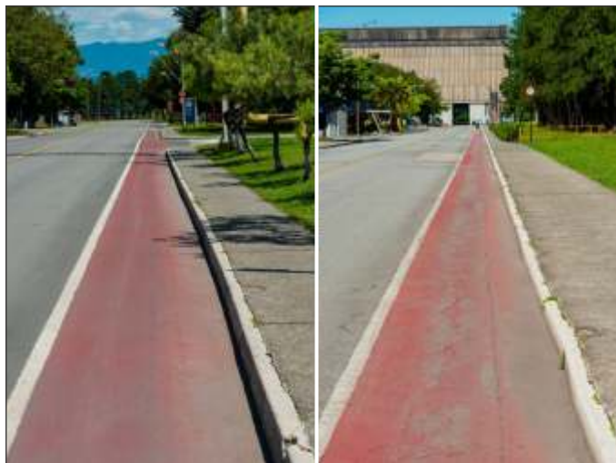
Figure 6: 7 months ageing (A1 – 0,05% Graphene) versus 6 months ageing (A2 – Reference).
