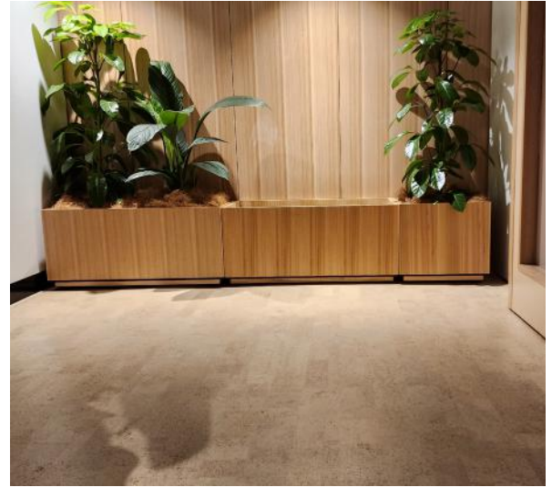
Photos of the Cork flooring installed in the ANZ trial program
