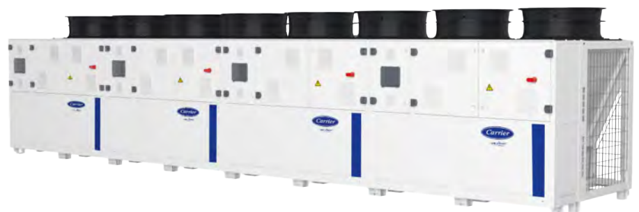
Four 120kW modular units, providing a combined 480 kW of heating capacity, were crane-lifted and installed on the hotel's rooftop
