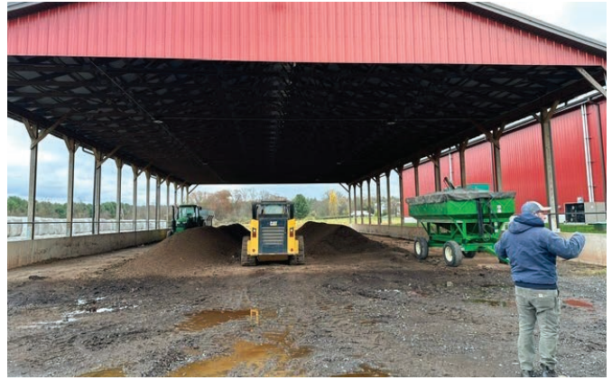
Steve Tomlinson explaining Carversville Farm Foundation's composting facility.
