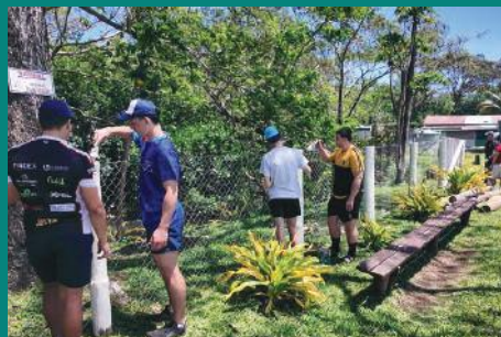
Hard at work repainting the fence at South Taveuni Secondary School.
