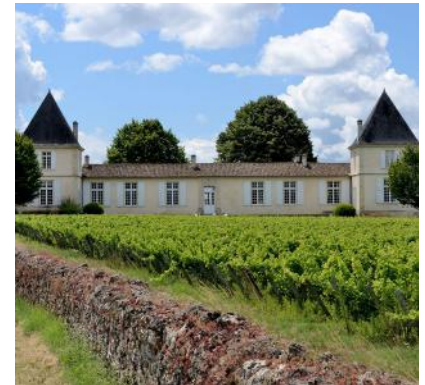
Château Climens - Winery
