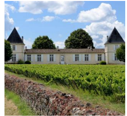
Château Climens - Winery
