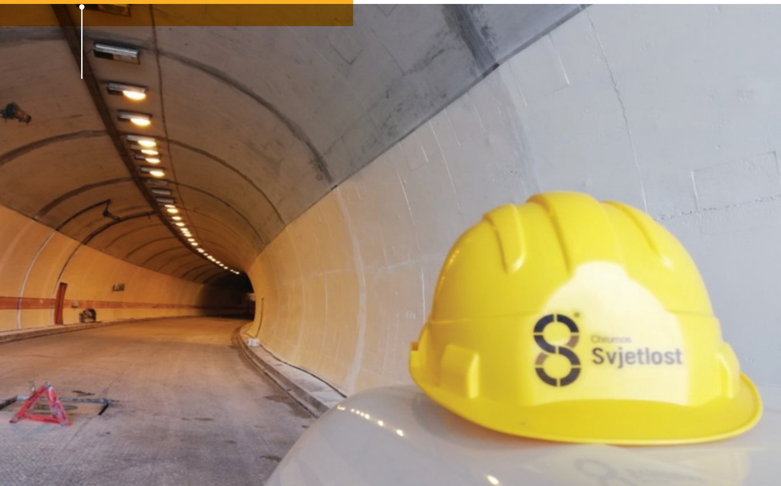
Mravince tunnel, works performed in 2019
