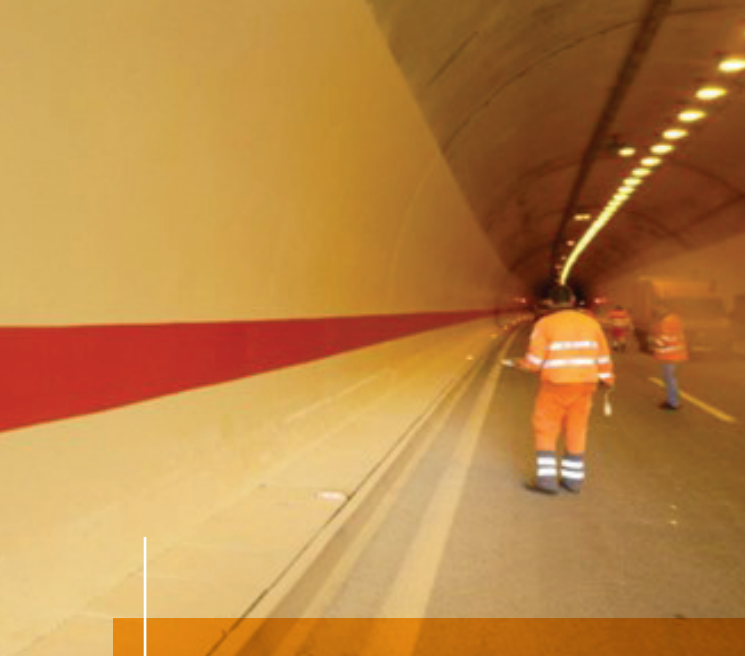
Work in the Brinje tunnel, 2019
