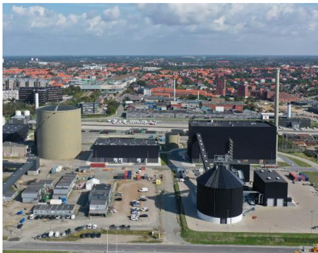
Above: Hot water storage tank, Mega Heat Pump hall and woodchip plant in the port of Esbjerg, Denmark. © DIN Forsyning.
