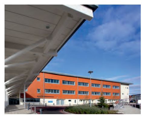
Heat pumps transform Tameside Hospital in £14m project P27
