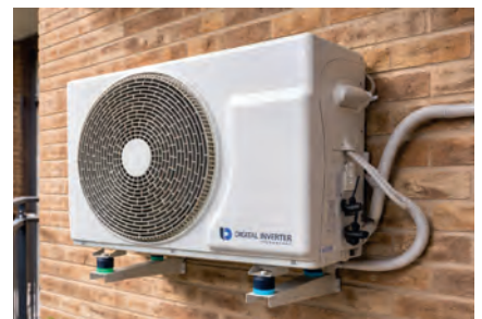
Outdoor units in residential settings require careful noise and vibration control
