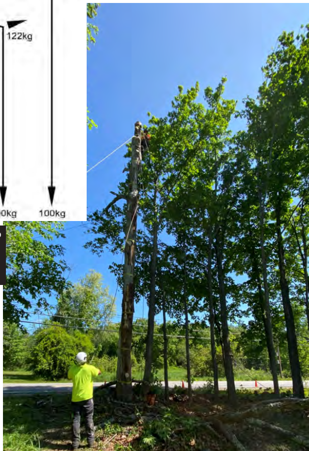
Photo 10- right: For that last piece, I decided to just put a tag line on it and pull it over without having to press my luck. We left the stem with the guy line attached
