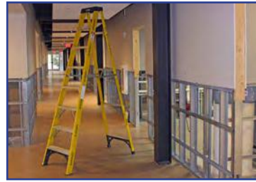
Vianney residence hall renovations complete.
