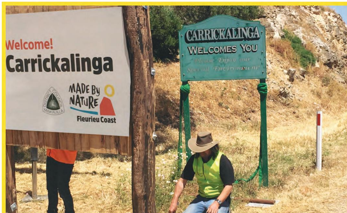
Image: The installation of the new signs.
